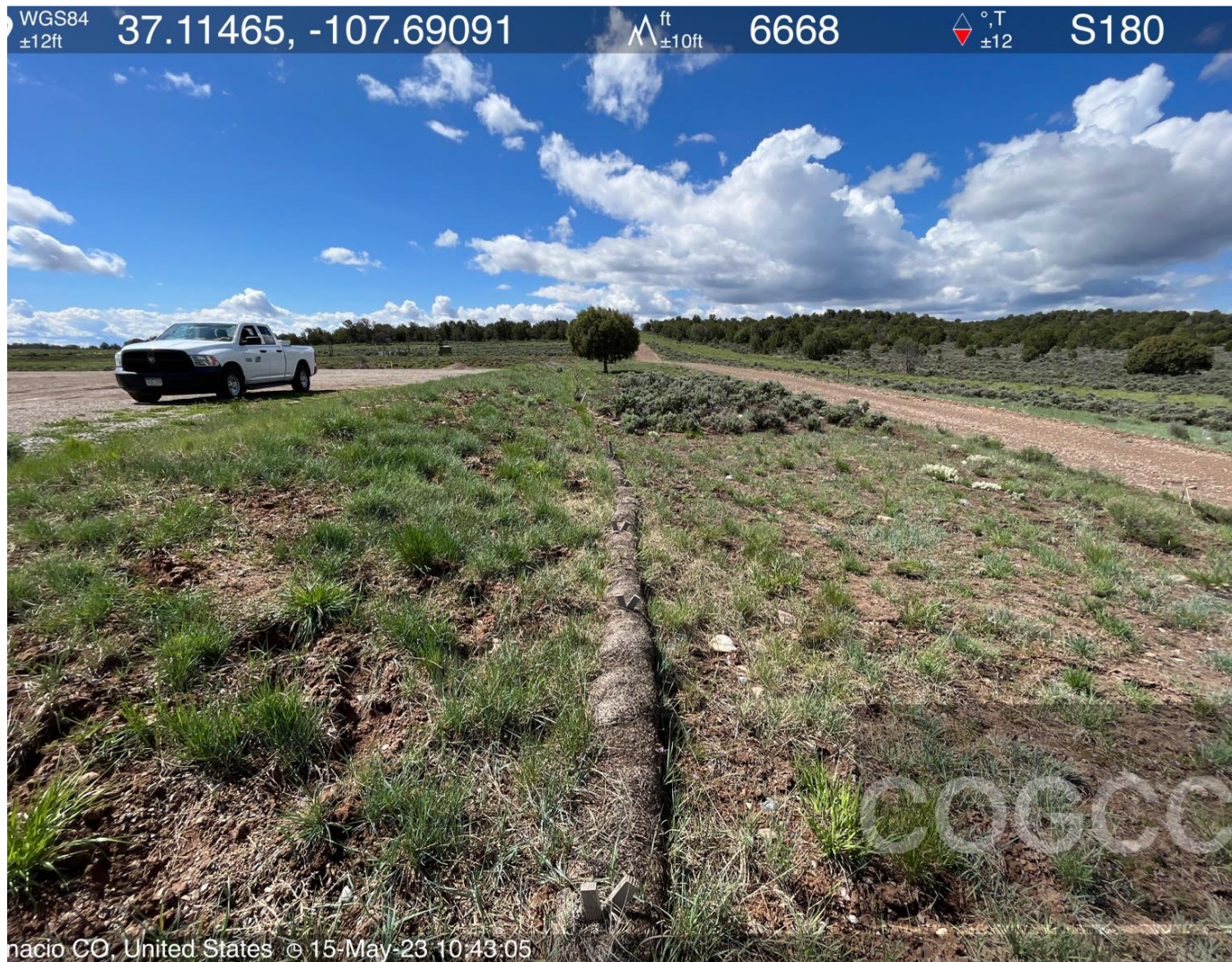
Photo #2. View of erosion wattles
