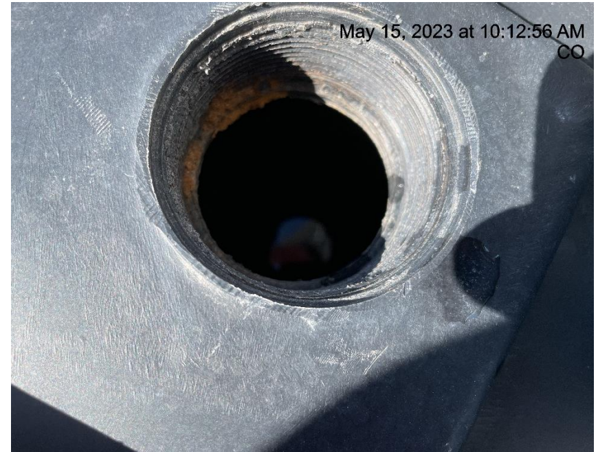
Photo # 7740 Chemical containment 7/8 th full/failure to maintain chemical BMP
