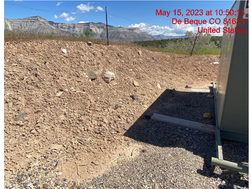
Berm Eroding onto Location – Photo #03356
