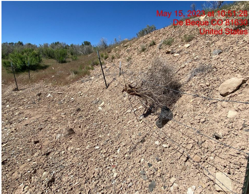
Berm Eroding onto Location – Photo #03361
