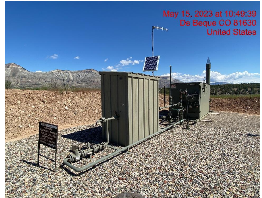
Gas Meter/Separator – Photo #03353
