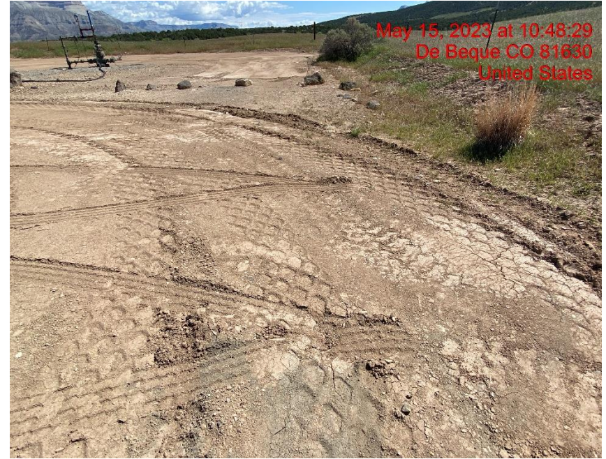
Location Lacks Stabilization – Photo #03350
