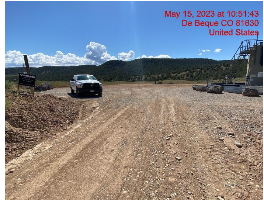
Insufficient Vehicle Tracking BMPs at Location Entrance/Exit – Photo #03362
