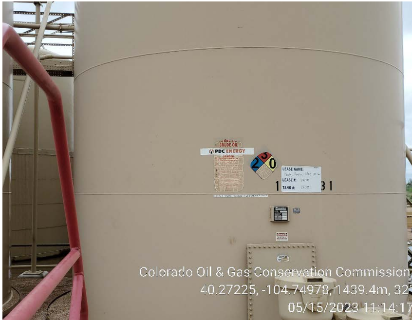
Crude oil tank placards and NFPA placard
