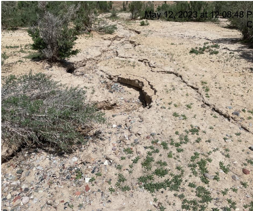
Photo # 7630 Erosion & transport of sediment/Insufficient run off controls/BMP's
