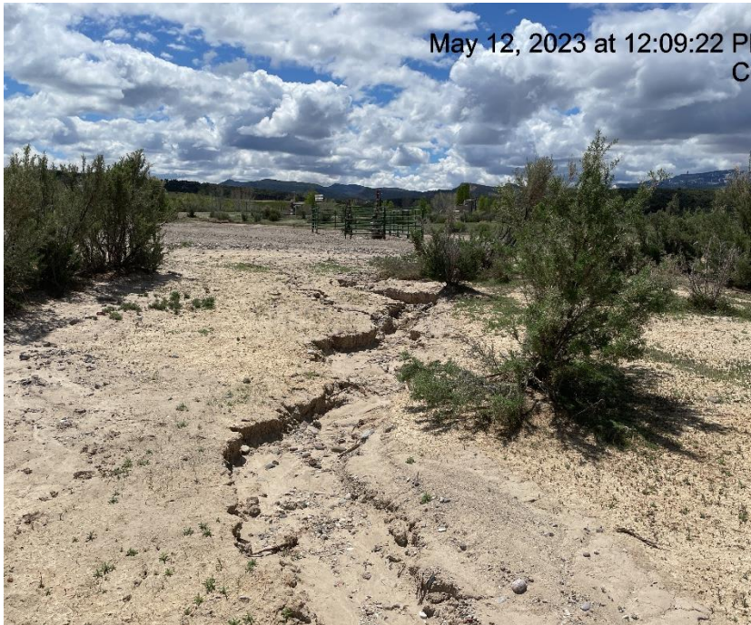
Photo # 7632 Erosion & transport of sediment/Insufficient run off controls/BMP's
