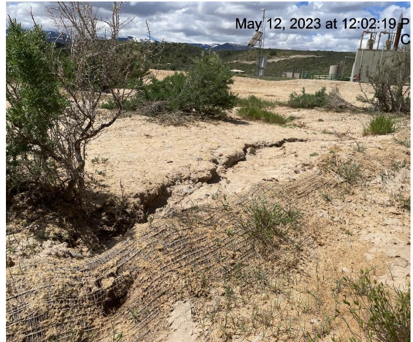
Photo # 7621 Erosion cutting into ditch
