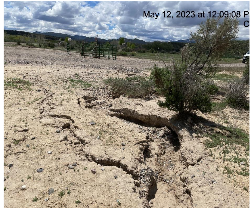
Photo # 7631 Erosion & transport of sediment/Insufficient run off controls/BMP's
