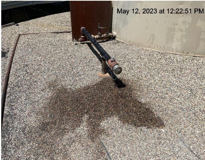
Photo # 7647 Stained gravel inside secondary containment
