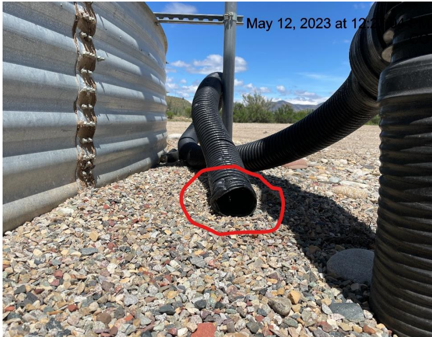
Photo # 7657 Flowline heating insulation open ended
