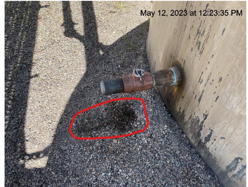
Photo # 7649 Stained gravel inside secondary containment
