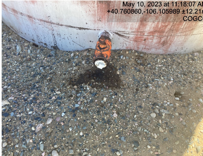
Staining under valve on tank
