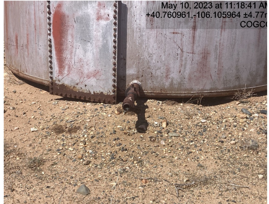
Valve on tank lacking plug/cap
