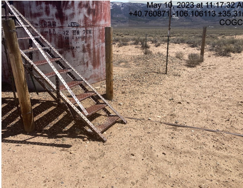
Insufficient secondary containment
