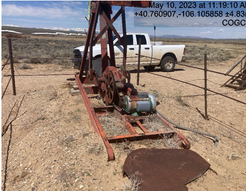
Pump jack is lacking guard
