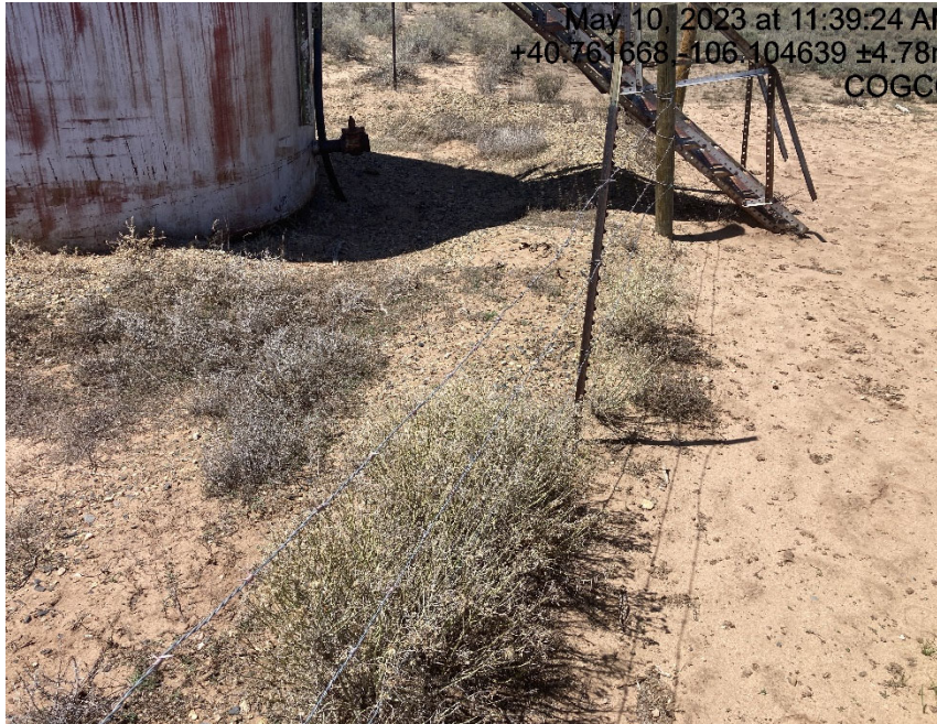
Insufficient secondary containment
