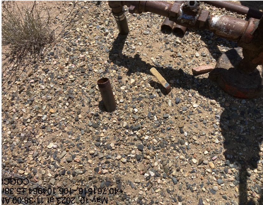
Casing valve. No Braden head access
