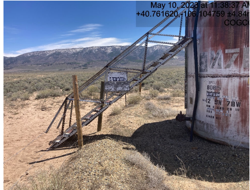
Tank battery lacking signage
