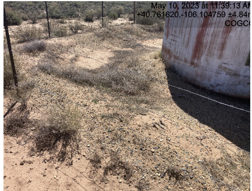
Insufficient secondary containment
