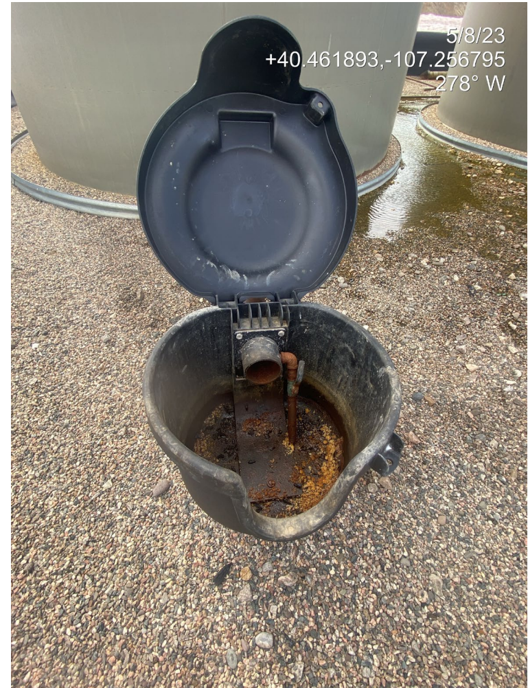
Photo 10. Photo shows a load line without a bull plug installed.
