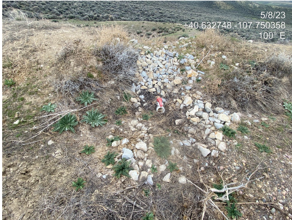
Photo 7. Photo taken from the east of the Location shows a drain pipe which leads through the fill slope. Stormwater is bypassing the drain and eroding the fill slope. Note also scotch and bull thistles.
