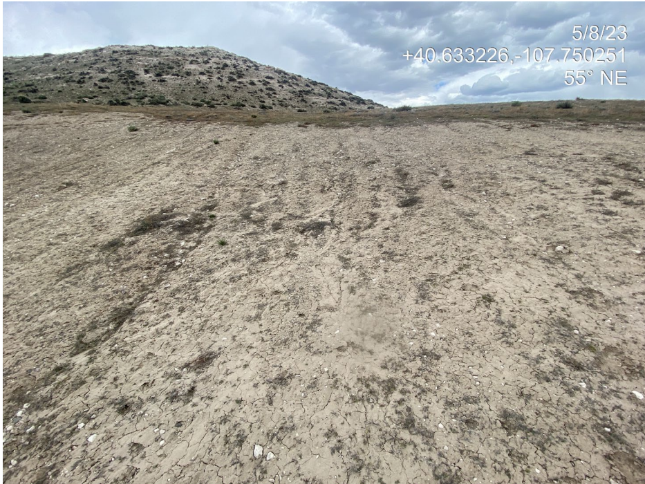
Photo 11. Photos taken at the northeast of the Location show rill erosion occurring on the unstabilized and unprotected cut slope. Photos also show Russian thistle, an undesirable plant species emerging.
