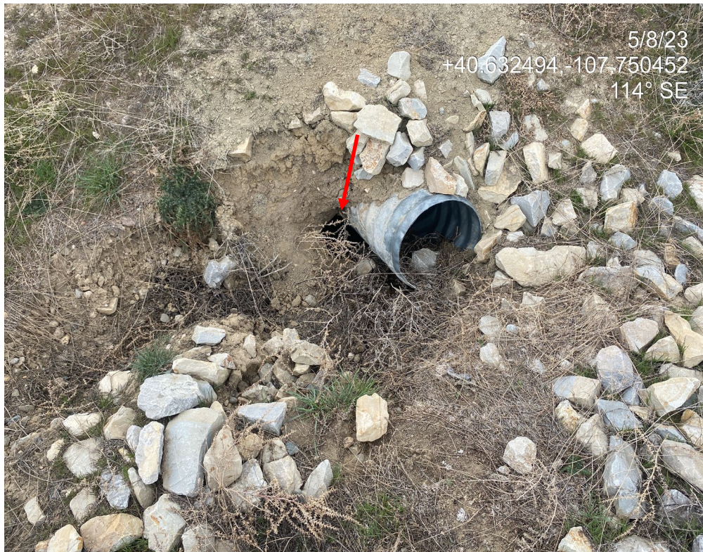
Photo 9. Photo taken from the fill slope at the southeast shows a fill slope drain. Stormwater is bypassing the drain and causing erosion. Photo left shows the inlet, right shows the outlet.
