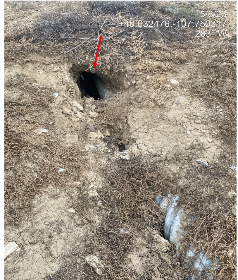
Photo 9. Photo taken from the fill slope at the southeast shows a fill slope drain. Stormwater is bypassing the drain and causing erosion. Photo left shows the inlet, right shows the outlet.
