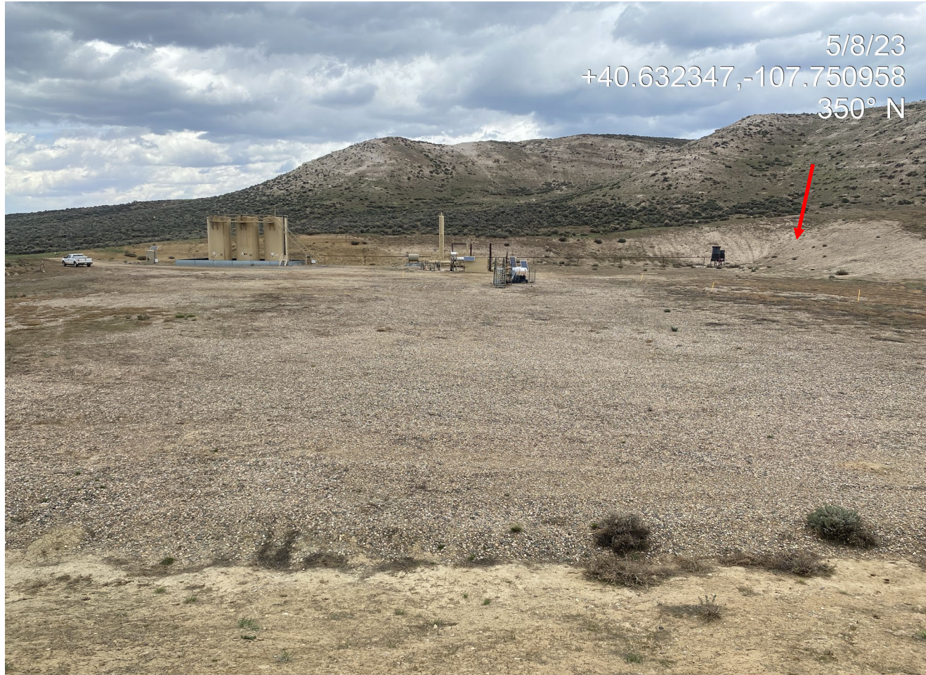
Photo 3. Photo taken from the south shows an overview of the location. Note the eroding cut slope (arrow).
