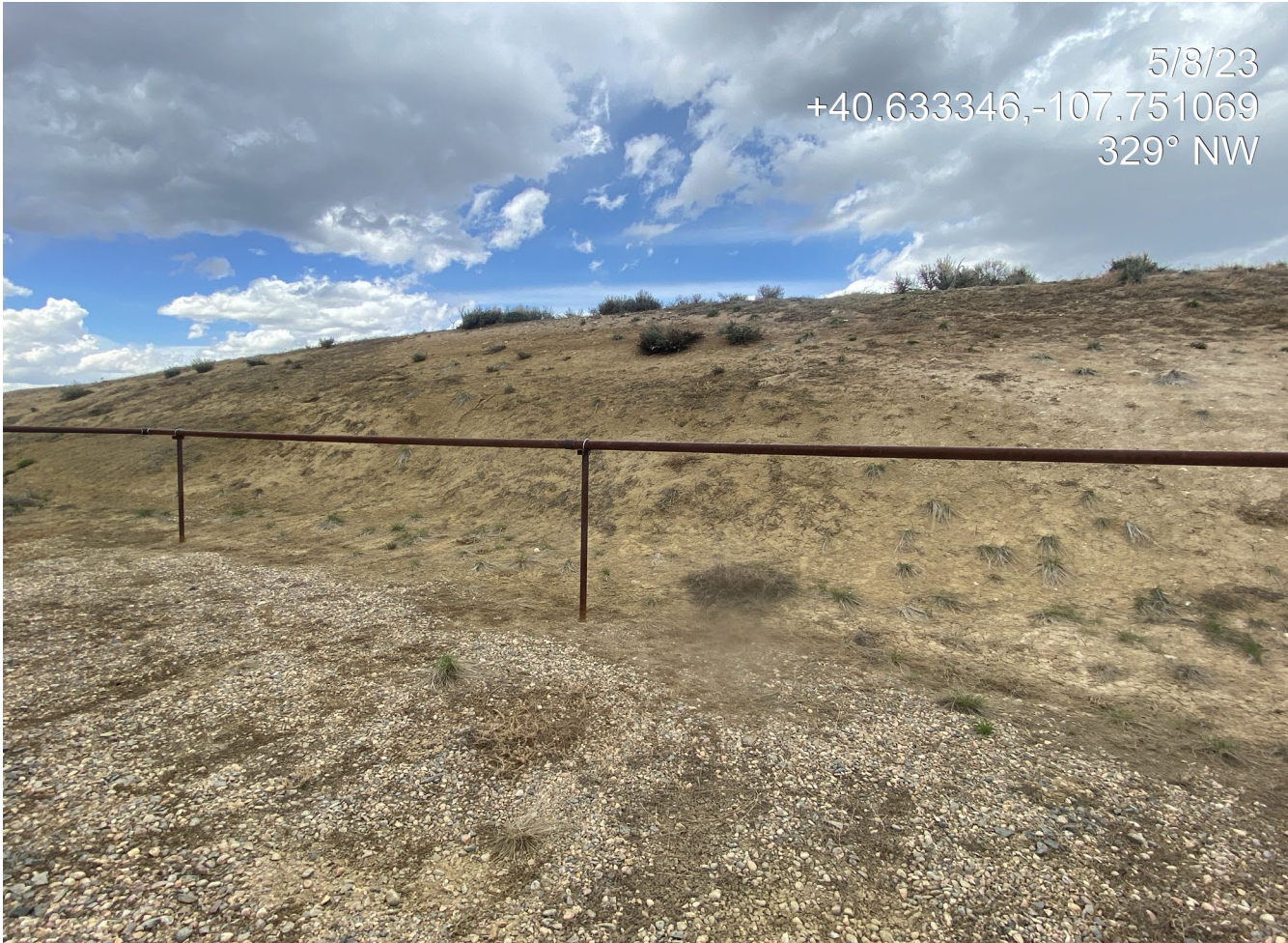
Photo 12. Photo taken at the north of the Location shows rill erosion occurring on the unstabilized and unprotected cut slope.
