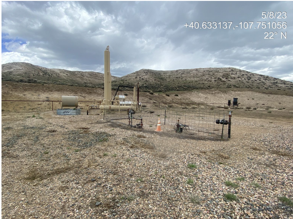
Photo 16. Photos show production areas to the north. Wildlife protection BMPs are missing/insufficient on the methanol tank secondary containment stock tank. The tank label is peeling and faded. Safety and identifying information is not legible.
