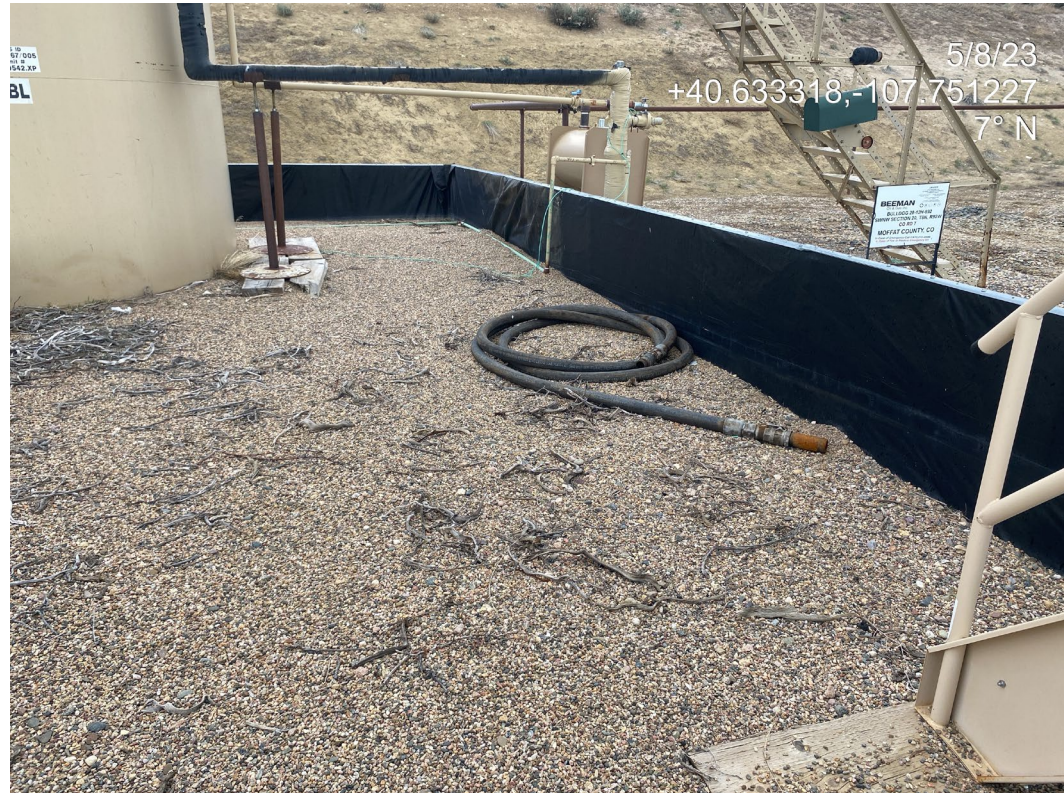
Photo 14. Photos show stained soils east of the tank battery (left) and unused hose equipment within the tank battery secondary containment berm (right).
