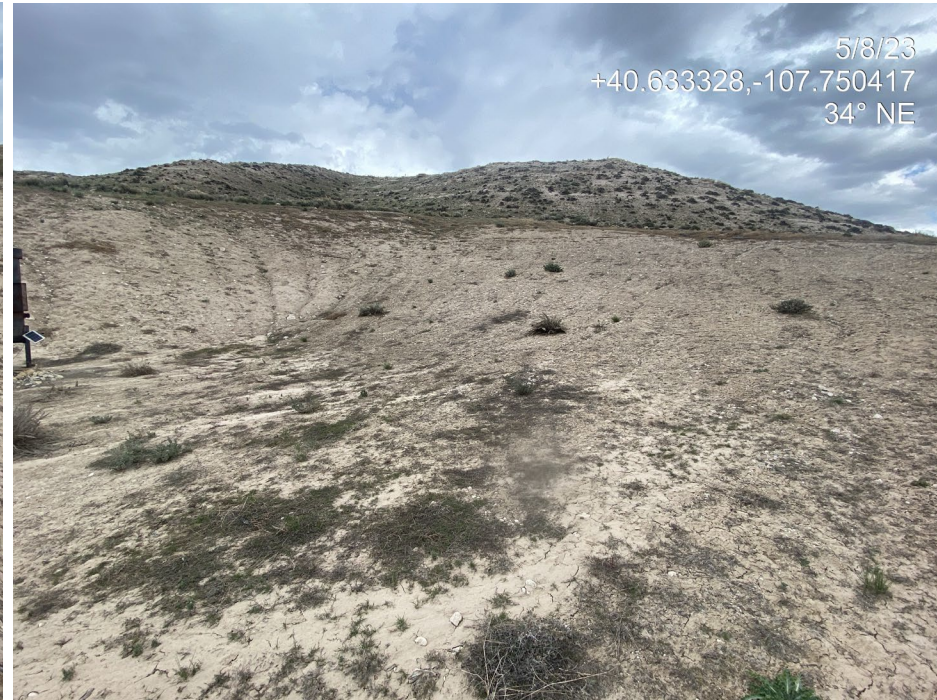
Photo 11. Photos taken at the northeast of the Location show rill erosion occurring on the unstabilized and unprotected cut slope. Photos also show Russian thistle, an undesirable plant species emerging.
