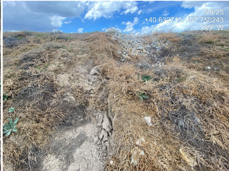
Photo 8. Photo taken from the east of the location shows where stormwater is bypassing a drain pipe and eroding the fill slope. Note the slope is densely colonized by noxious weeds and undesirable plant species.
