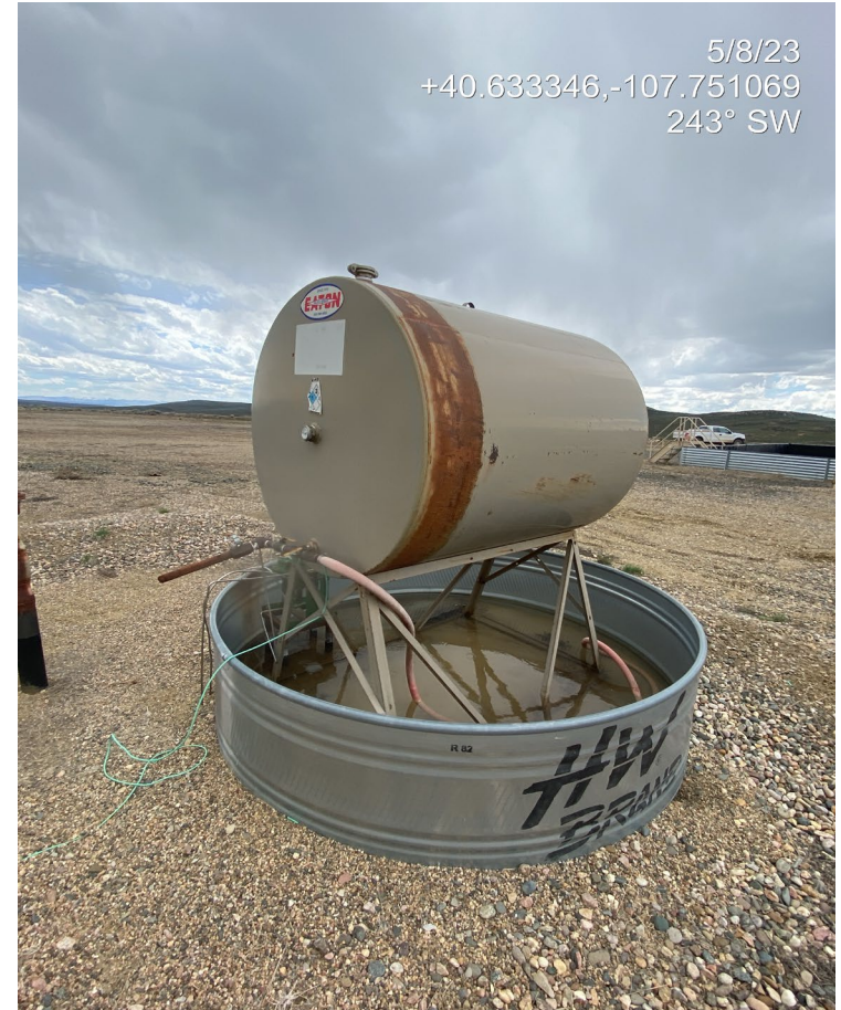
Photo 16. Photos show production areas to the north. Wildlife protection BMPs are missing/insufficient on the methanol tank secondary containment stock tank. The tank label is peeling and faded. Safety and identifying information is not legible.
