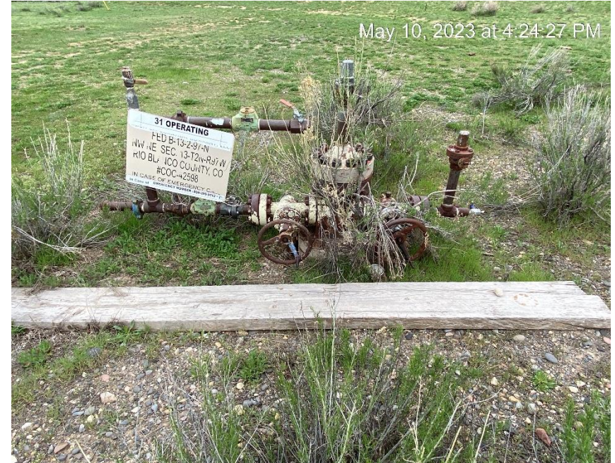
Sign and wellhead
