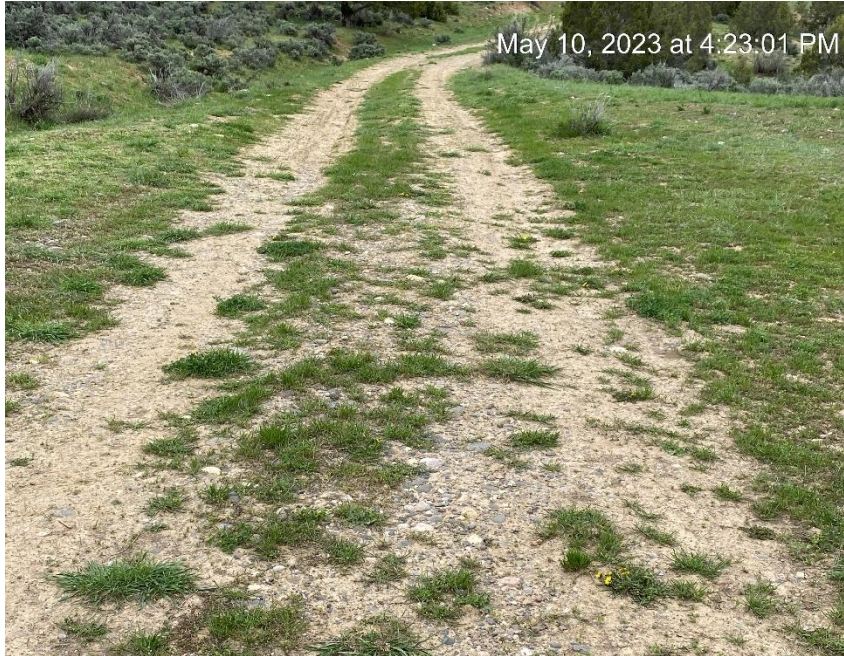
Access road at location
