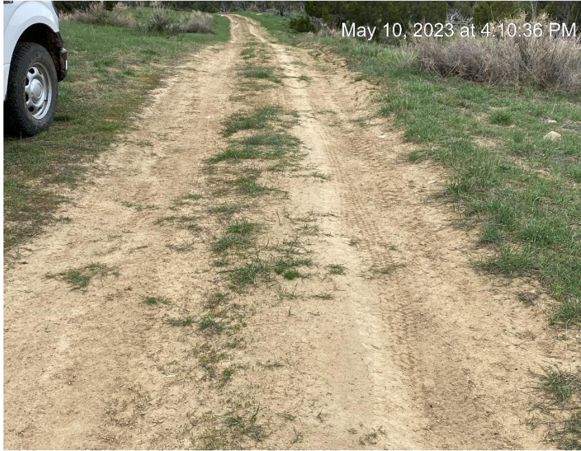
Access road at location
