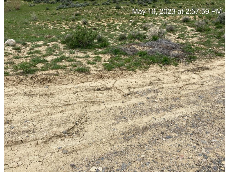
Erosion and sediment migration from alternate entrance to location
