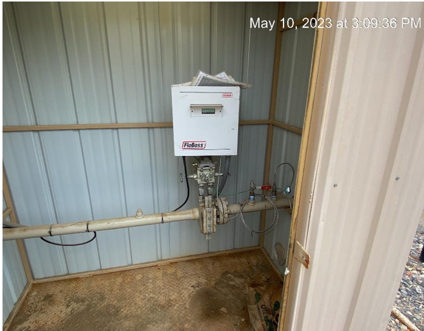
Gas meter calibration card not visibly displayed
