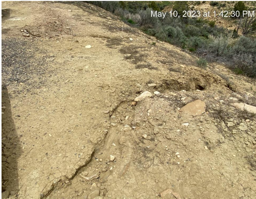
Erosion and soil migration
