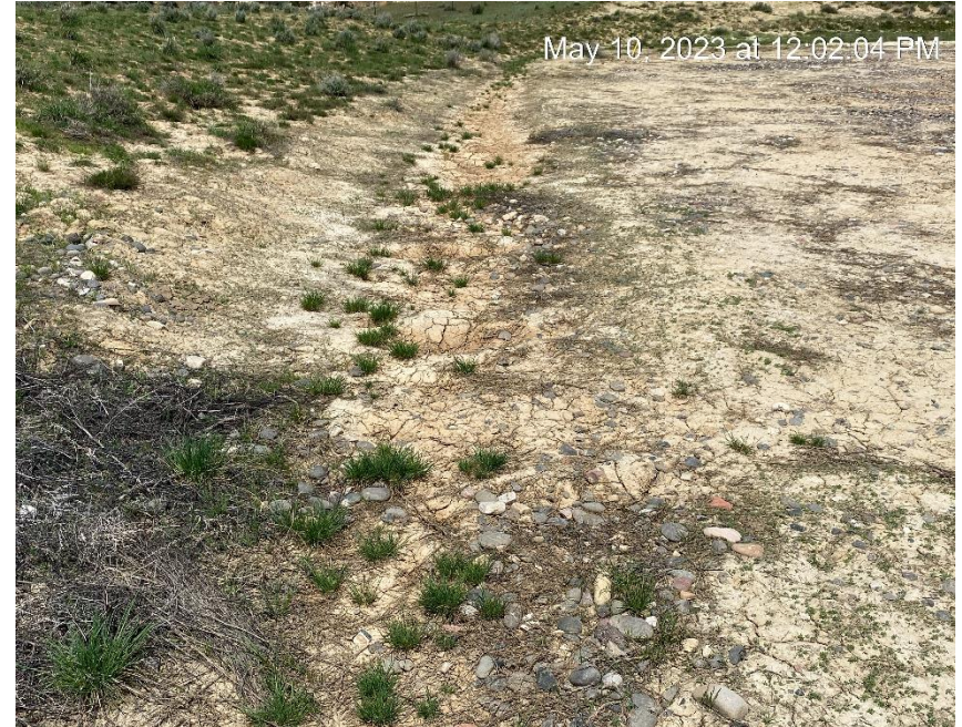
Diversion ditch full of sediment
