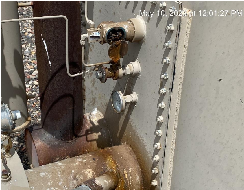
Oil leak on crude oil tank
