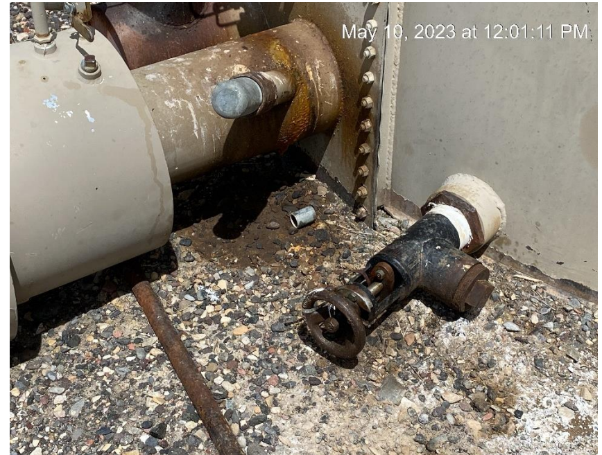
Soil staining from leak on crude oil tank
