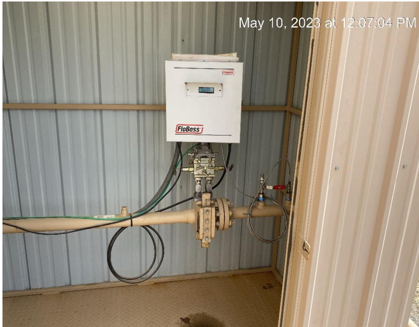
No visible display of gas meter calibration
