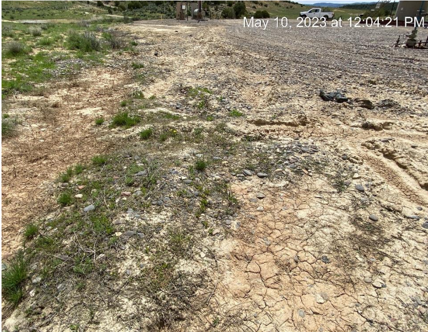
Diversion ditch damage and full of sediment
