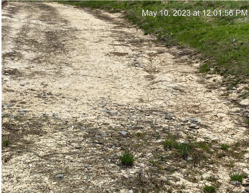
Bare slope and sediment migration off location
