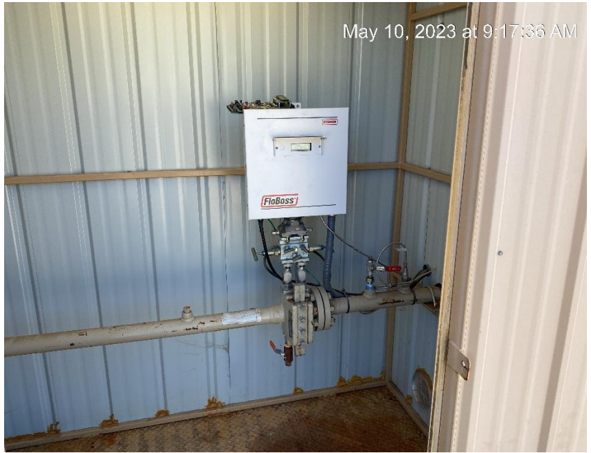
Gas meter calibration not visibly displayed
