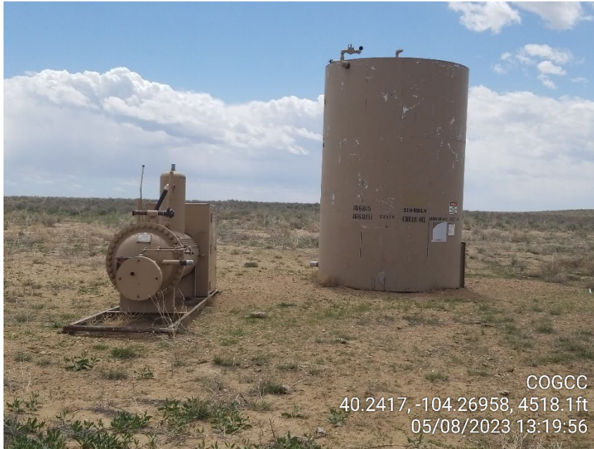
Photo 1 – Separator and Tank
