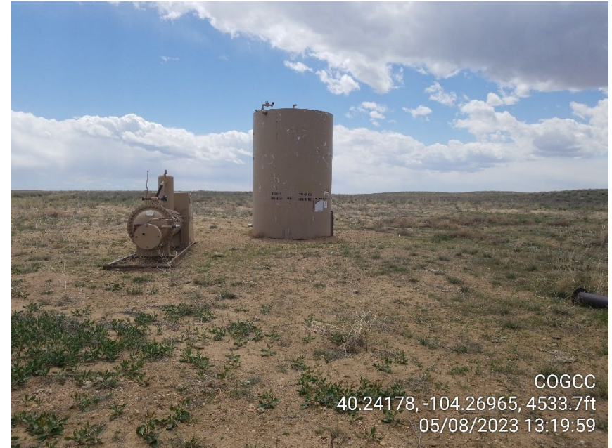
Photo 2 – Separator and Tank
