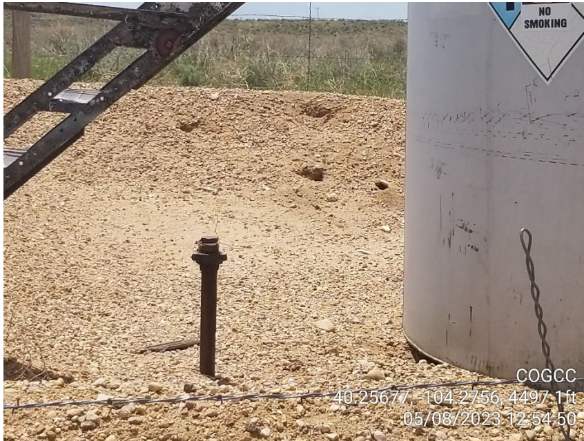
Photo 5 – Unmarked Riser
