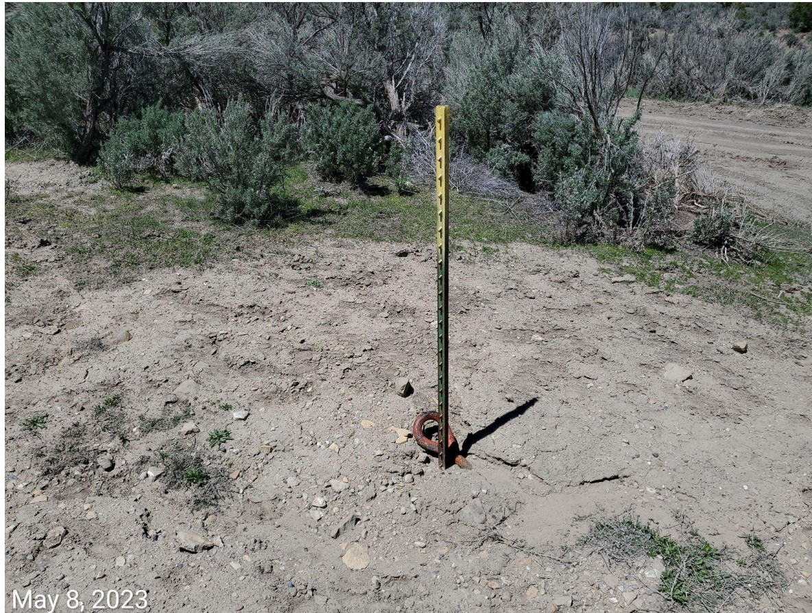
Photo 5: Photo example showing anchors marked on Location.
