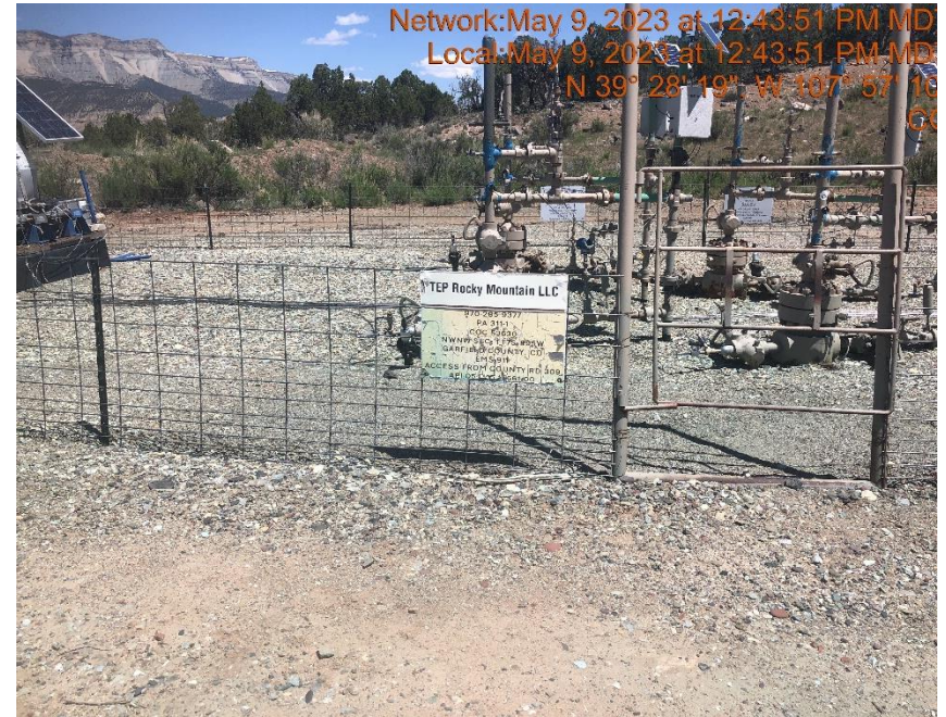
Photo #9899 Multiple wellhead signs weathered and not legible.
