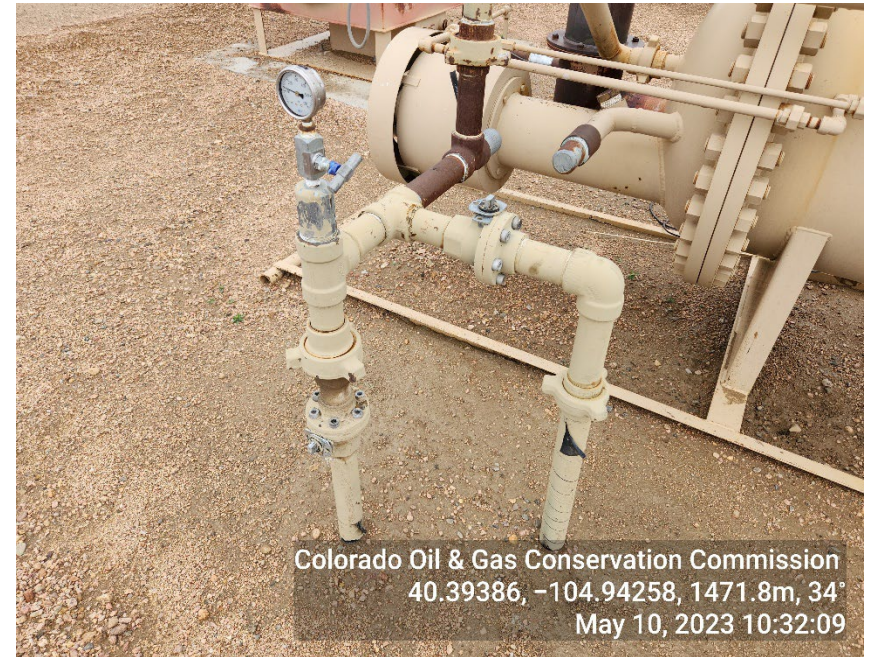
Photo 4: Valves appear to be open, pressure is present on gauge
