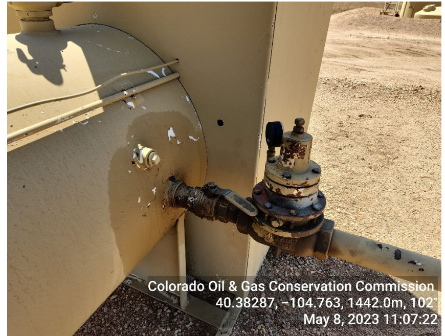
Photo 8: Valve appears to be open
