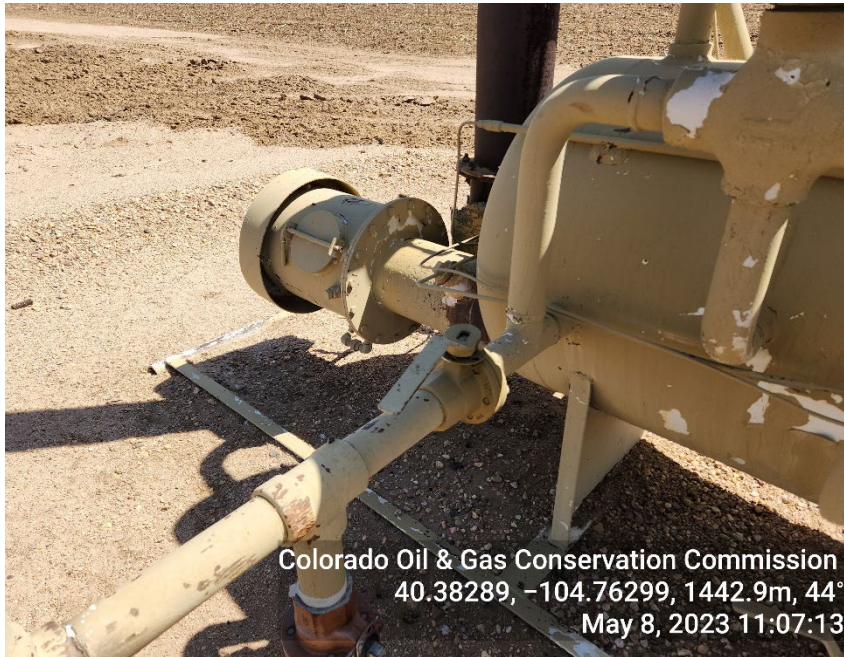
Photo 7: Valve appears to be open
