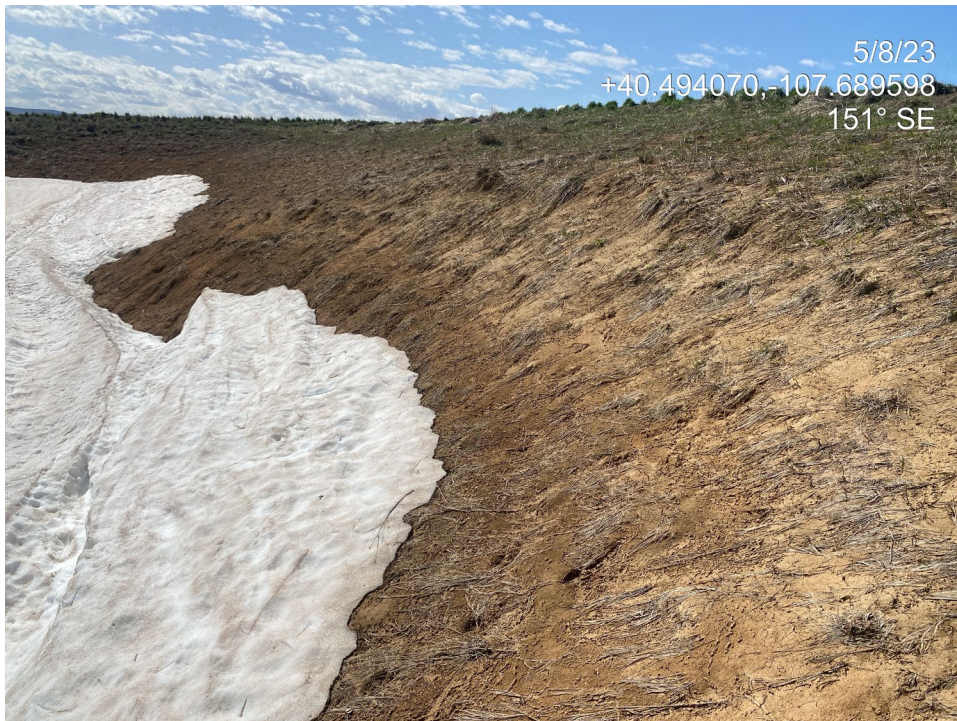
Photo 4. Photos shows unstabilized cut slopes at the west of the location.
