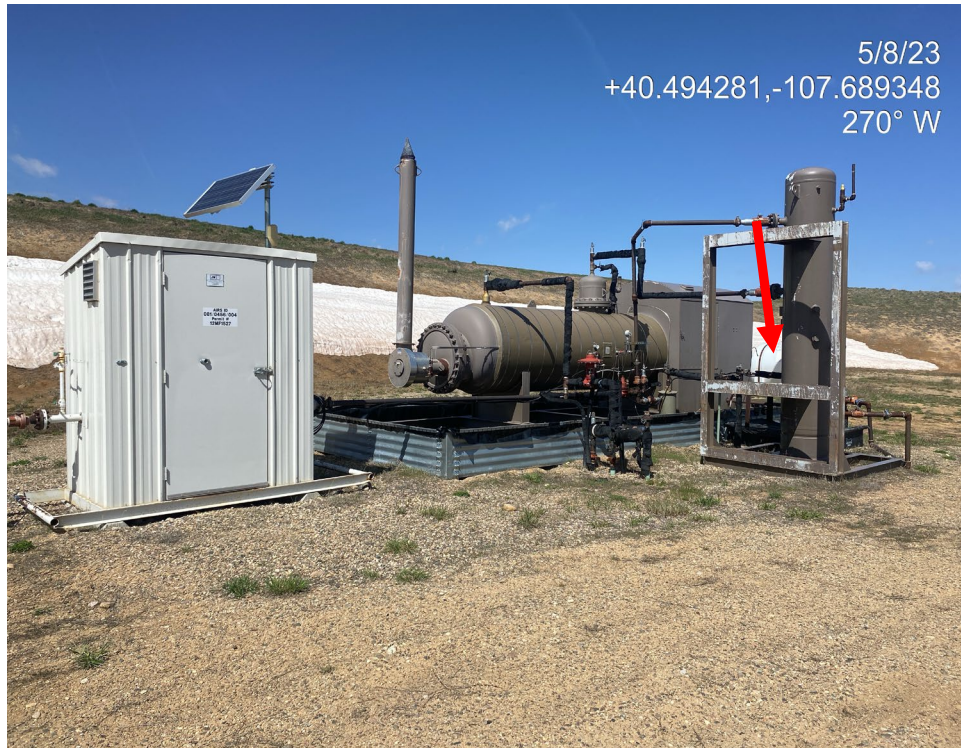
Photo 10. Photos show production areas. The secondary containment device for the methanol tank adjacent to the separator is bent and not in proper functioning condition to contain a spill.
