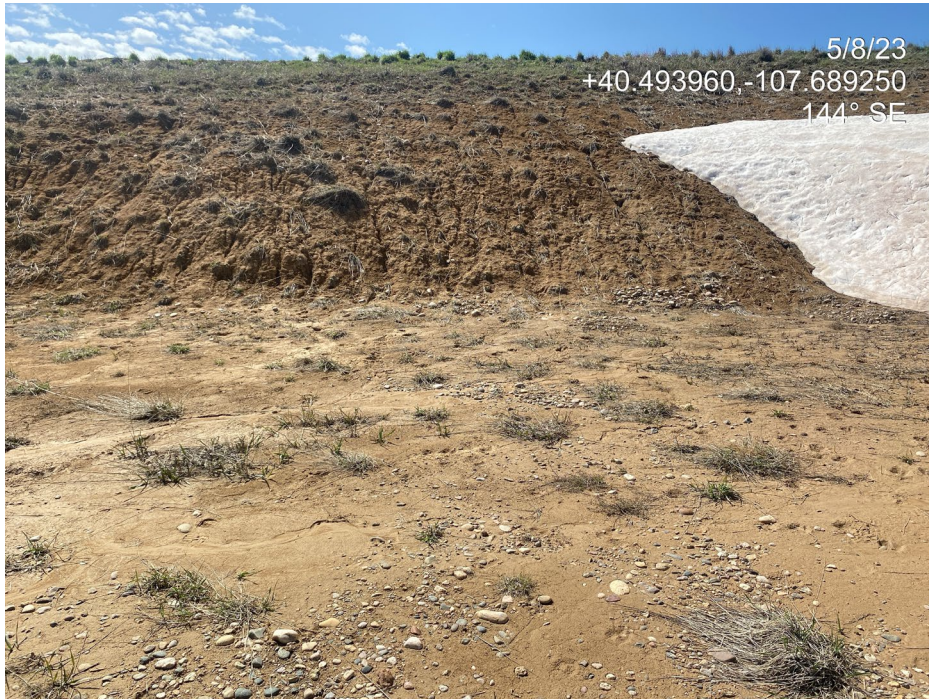
Photo 5. Photos shows unstabilized cut slopes at the southwest of the location.
