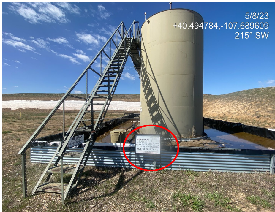
Photo 7. Photos show production areas. The tank battery sign (circled) does not comply with Rule 605.e and is partially illegible.
