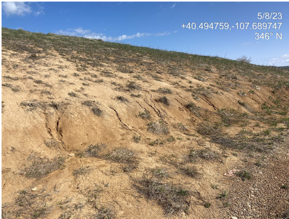
Photo 2. Photos show rill erosion on unstabilized cut slopes at the north of the Location.
