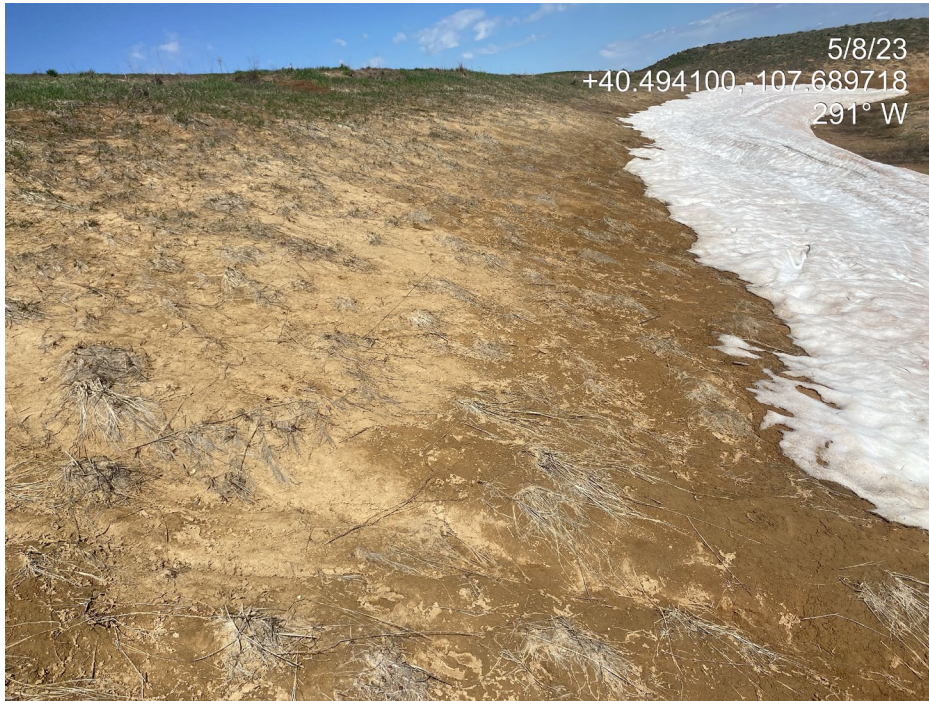
Photo 3. Photos show unstabilized cut slopes at the west of the location.
