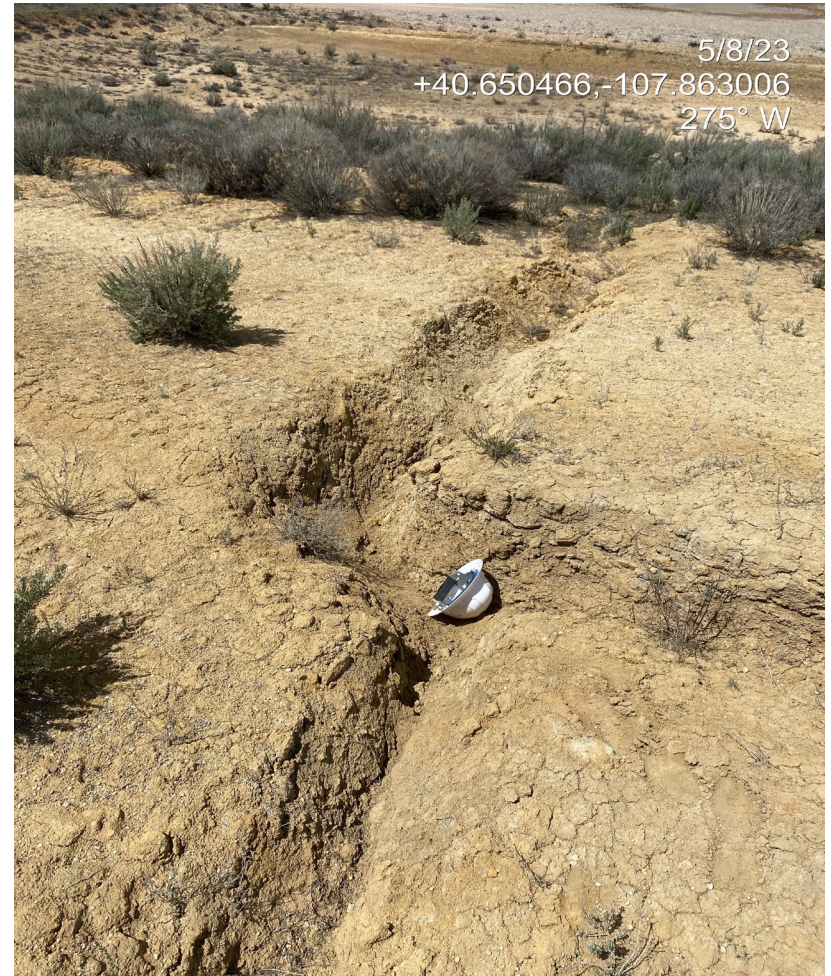
Photo 5. Photo shows gully erosion on the cut slope to the east.
