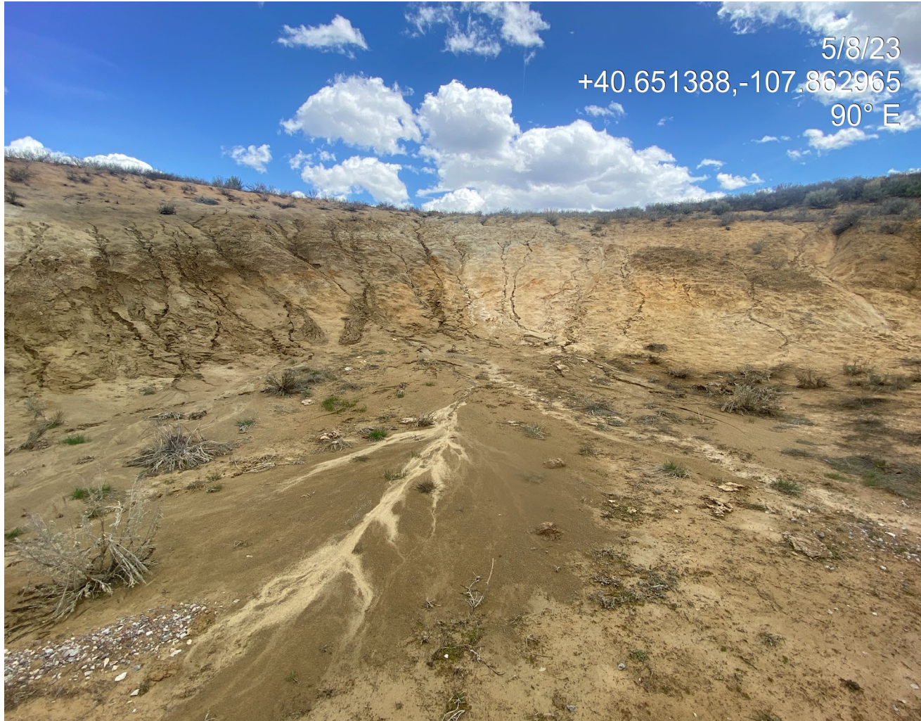
Photo 7. Photo shows rill erosion on the unstabilized cut slope to the northeast.
