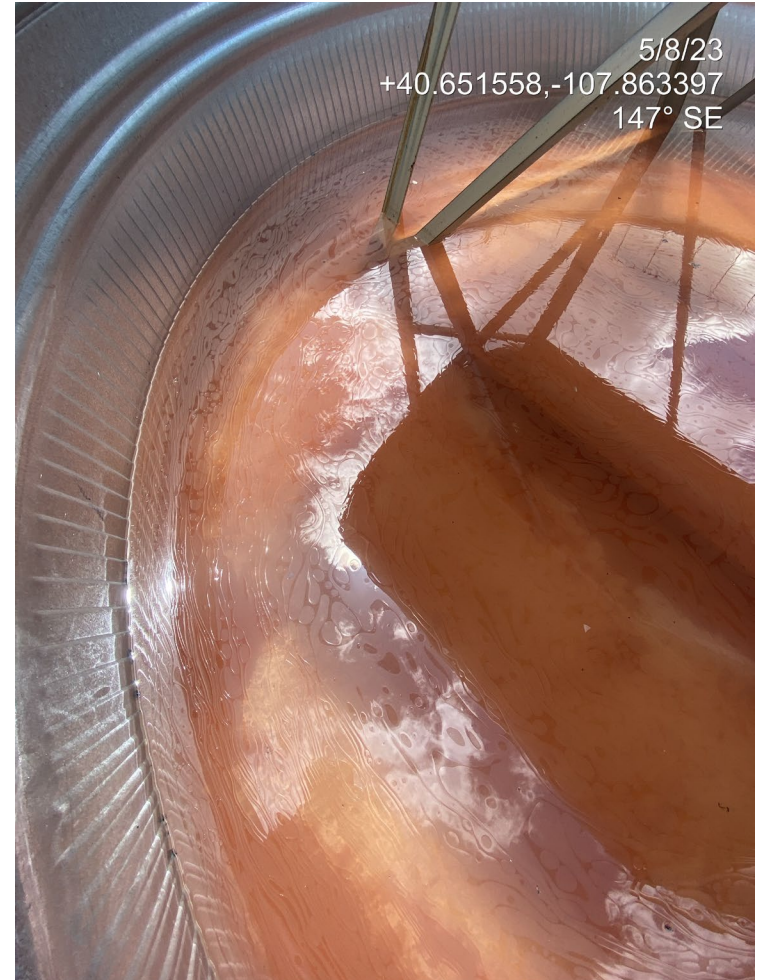
Photo 9. Photos show a methanol tank at the north of the Location lacks wildlife protection BMPs on the secondary containment stock tank. Photos also shows impacted fluid within secondary containment.
