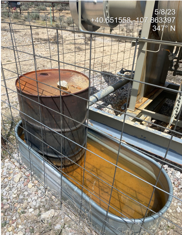
Photo 10. Photo taken to the north shows inadequate wildlife protection BMPs on the secondary containment stock tank.
