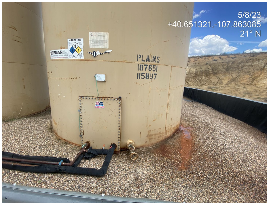
Photo 13. Photos show staining below a crude oil tank, which appears to be leaking.
