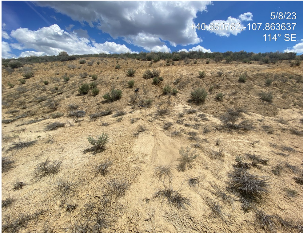
Photo 6. Photos show rill erosion on the unstabilized cut slope.
