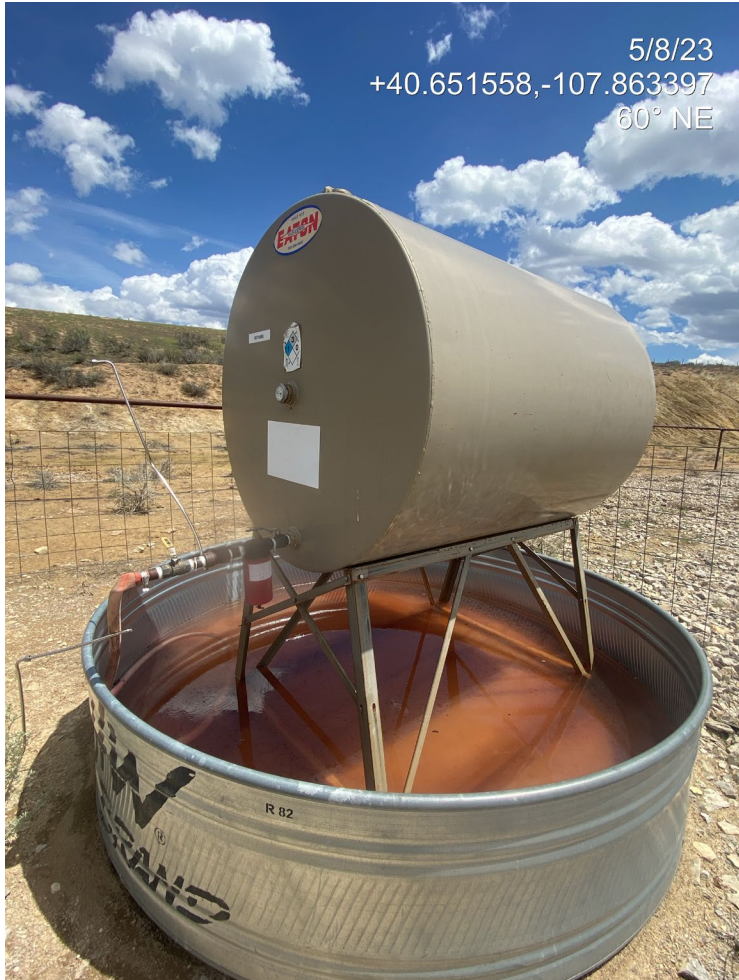
Photo 9. Photos show a methanol tank at the north of the Location lacks wildlife protection BMPs on the secondary containment stock tank. Photos also shows impacted fluid within secondary containment.
