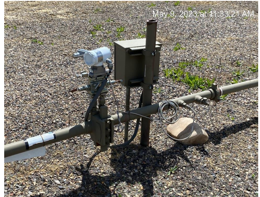
Gas meter calibration card not visibly displayed. WRD Wyatt 25-44W
