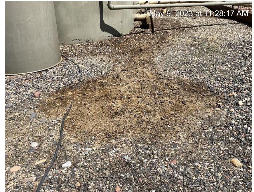
Soil staining inside tank battery containment
