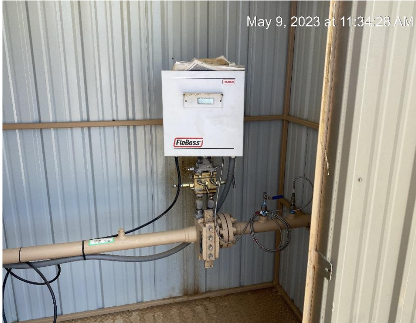
Gas meter calibration card not visibly displayed. WRD Wyatt 25-44.
