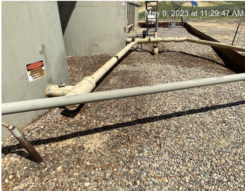
Soil staining inside tank battery containment
