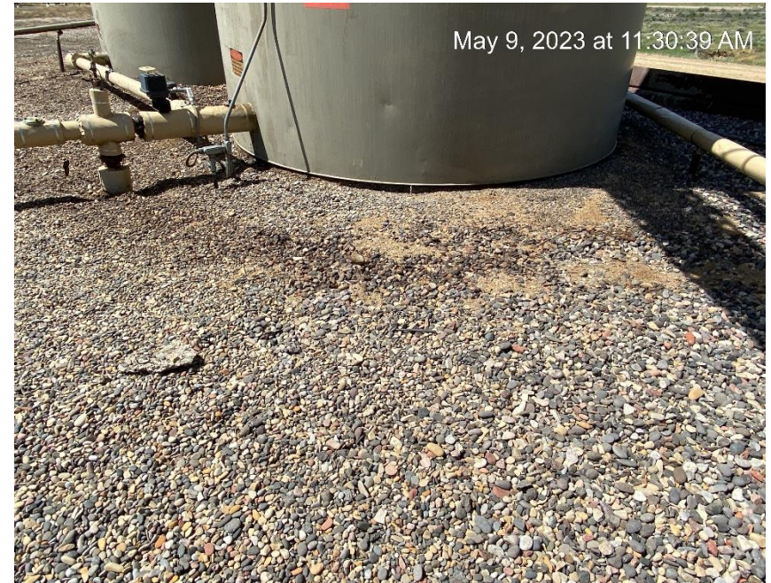
Soil staining inside tank battery containment
