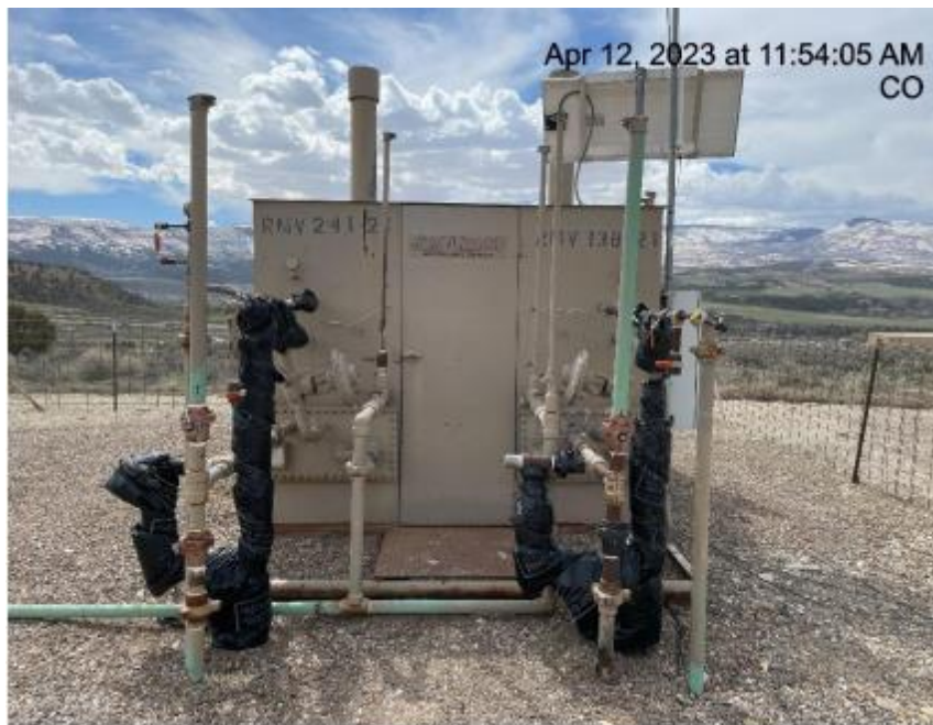
Photo # 5126 From Inspection 708900271 conducted on 04/12/2023 Meter calibration info not conspicuously posted
