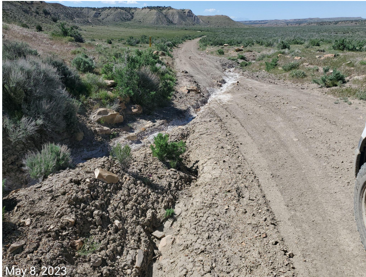
Photo 7: Gully erosion along access road. BMPs to manage runoff remain missing or insufficient.
