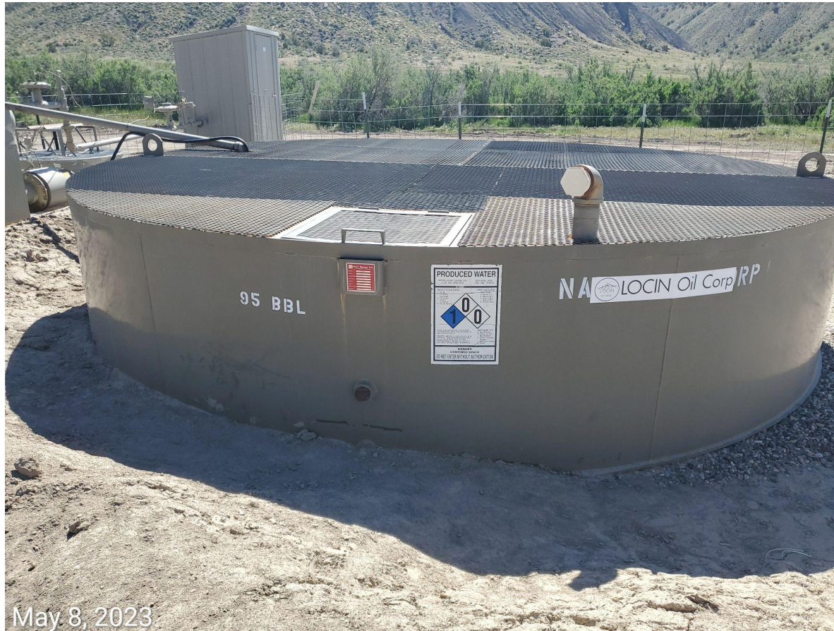
Photo 5: Tank battery on south end of the Location. Signage on tank does not comport with 605 Rules.
