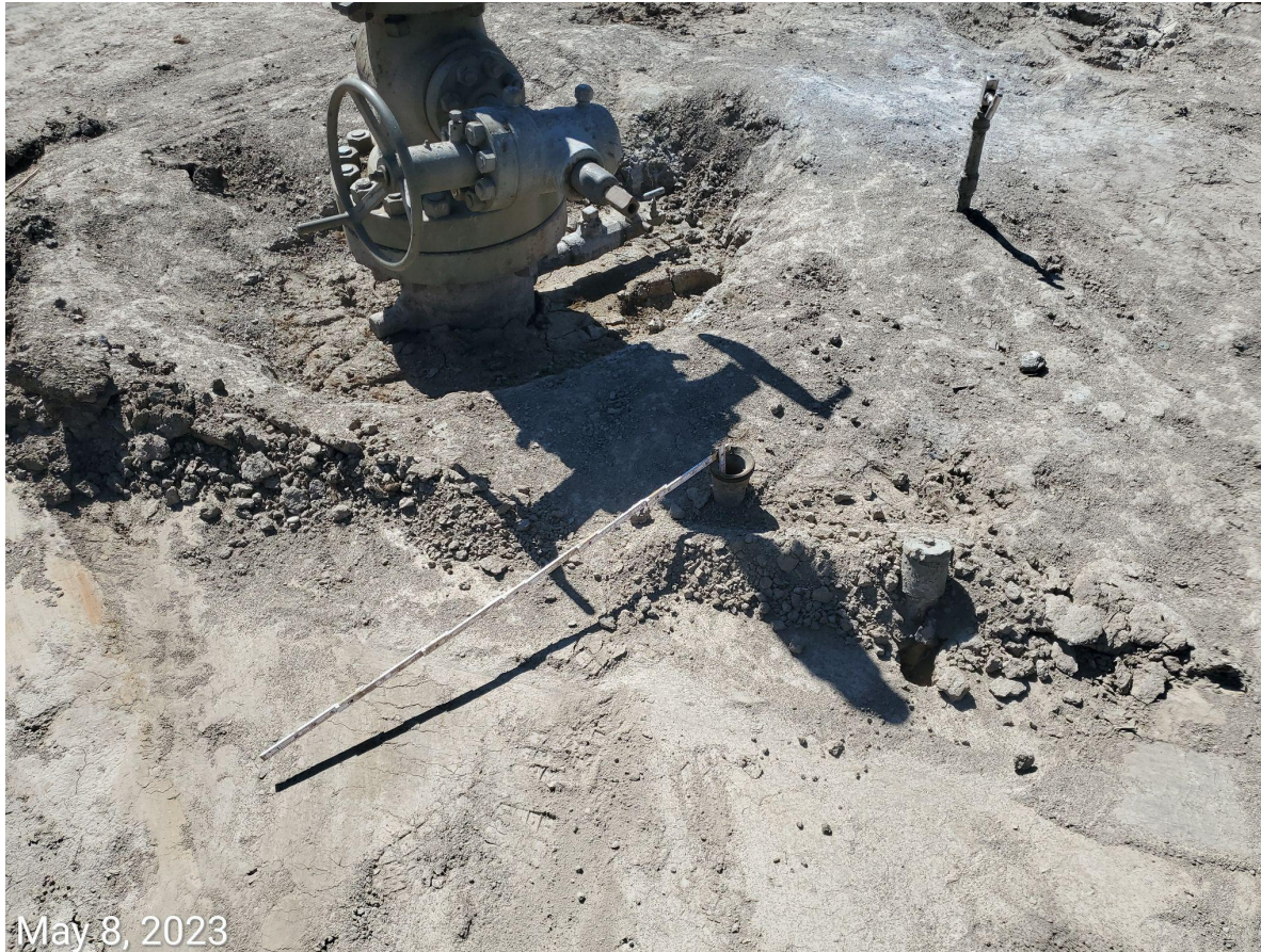
Photo 7: Riser adjacent to well has not been properly capped, and remains exposed.
