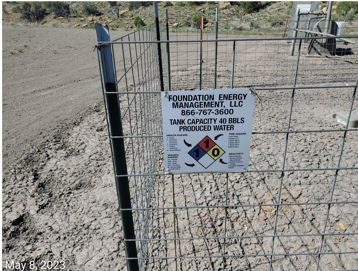
Photo 3: Signage at battery facility/tank remains inaccurate. Labels not observed on partially buried tank. Signage at battery does not comport with Rules 605.e and 605.h
