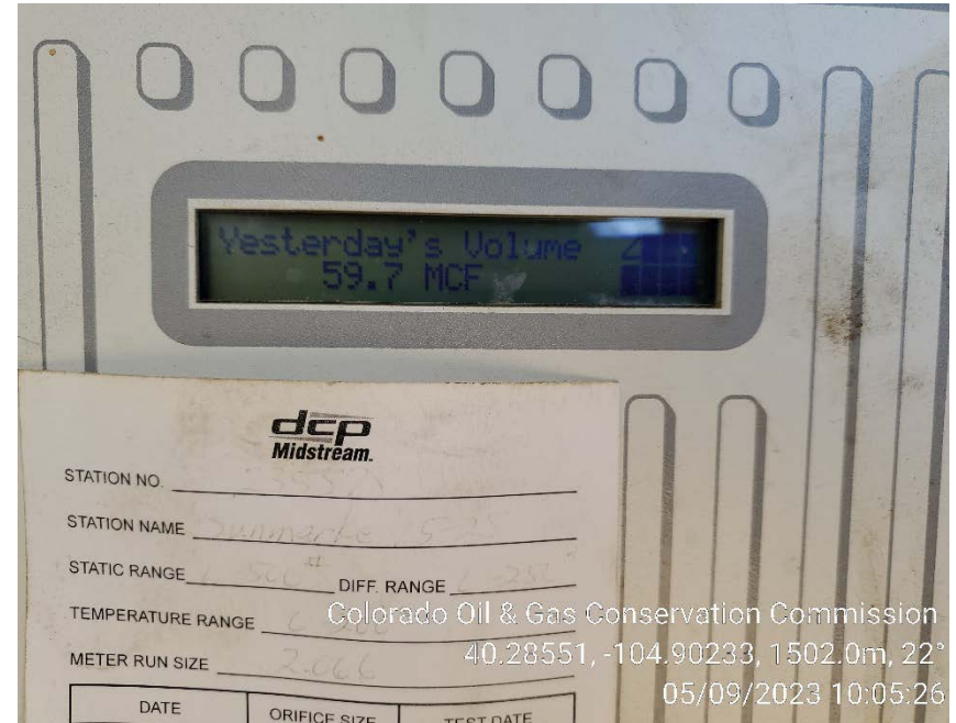
DCP meter station calibration card and previous day product sold volume
