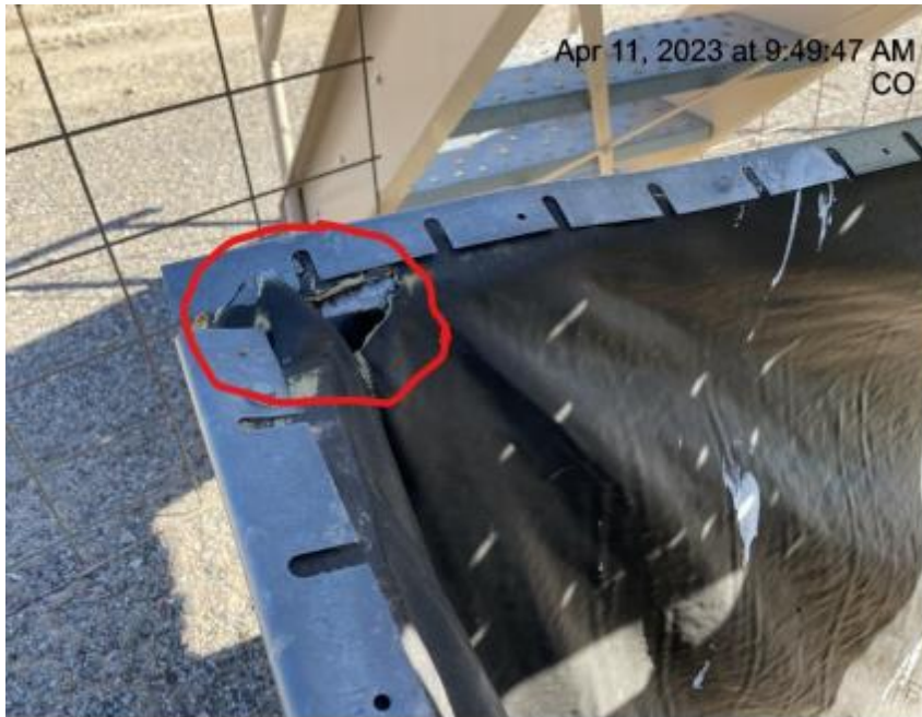
Photo # 4958 From Inspection 708900261 conducted on 04/11/2023 Containment liner needs maintenance
