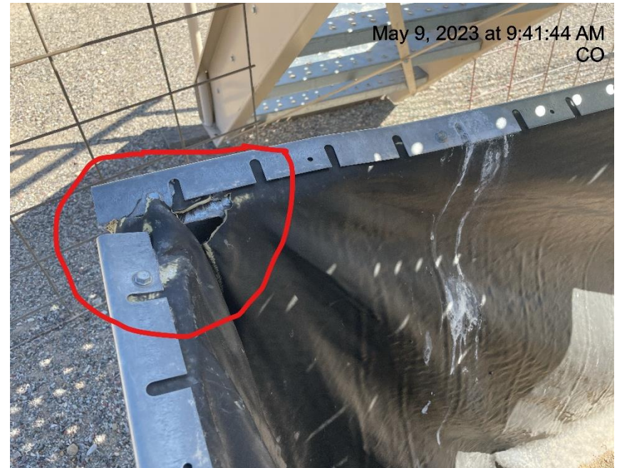
Photo # 7247 Containment liner needs maintenance
