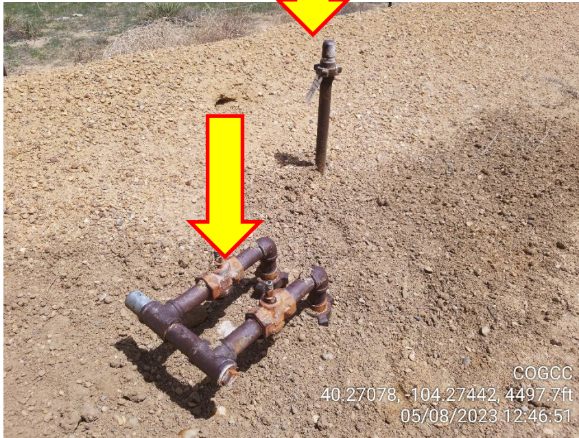
Photo 9 – Unmarked Risers in Tank Berm
