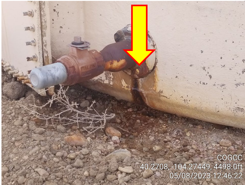
Photo 7 – Back Drain Valve on Produced Water Tank
