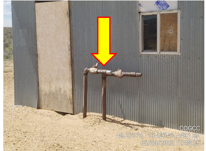
Photo 16 – Unmarked Risers
