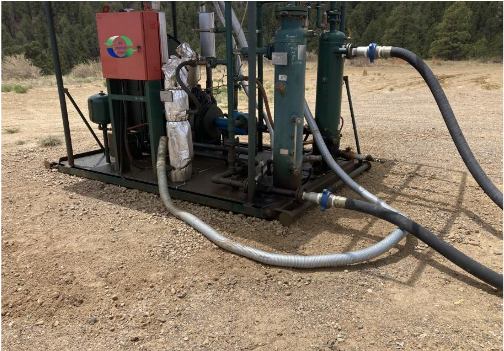
PHOTO 1: THE OILY FLUID FROM THE SKID HAS BEEN REMOVED AND PROPERLY DISPOSED OF. MAINTENANCE HAS BEEN PERFORMED AND THE SELF INSPECTION PROCESS REVIEWED.
