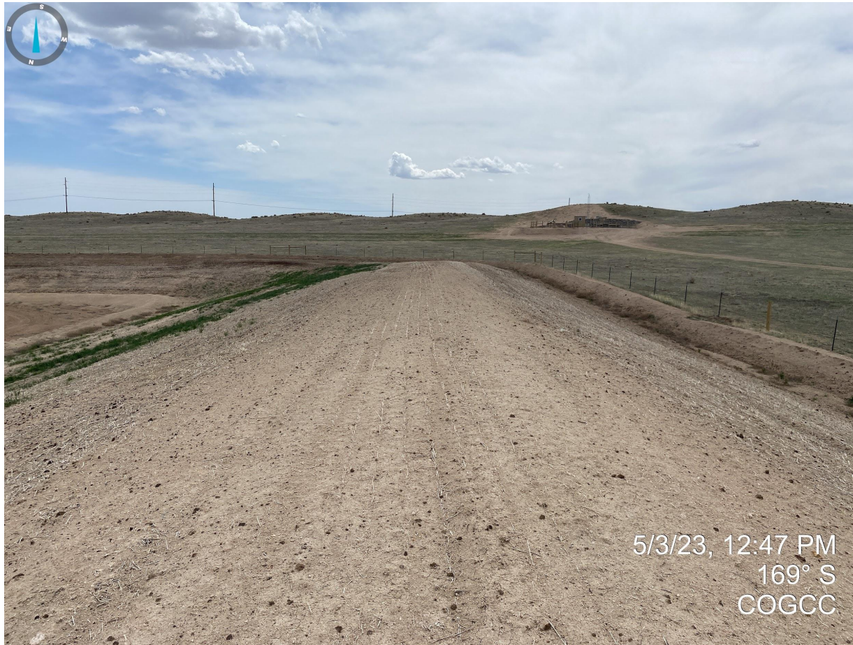
Photo 12. From top of stockpile; see comments in Photo 8.
