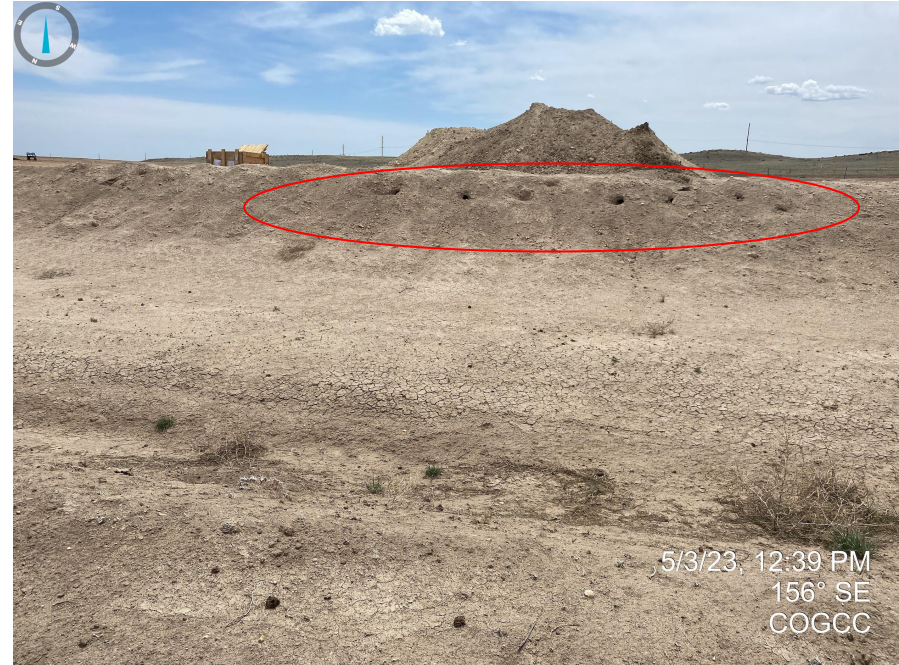
Photos 3 & 4. Rill erosion at culvert (left) and animal burrows in the interior stormwater berm (right); see comments in Photos 1 & 2 for additional information.
