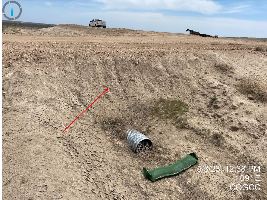
Photos 3 & 4. Rill erosion at culvert (left) and animal burrows in the interior stormwater berm (right); see comments in Photos 1 & 2 for additional information.
