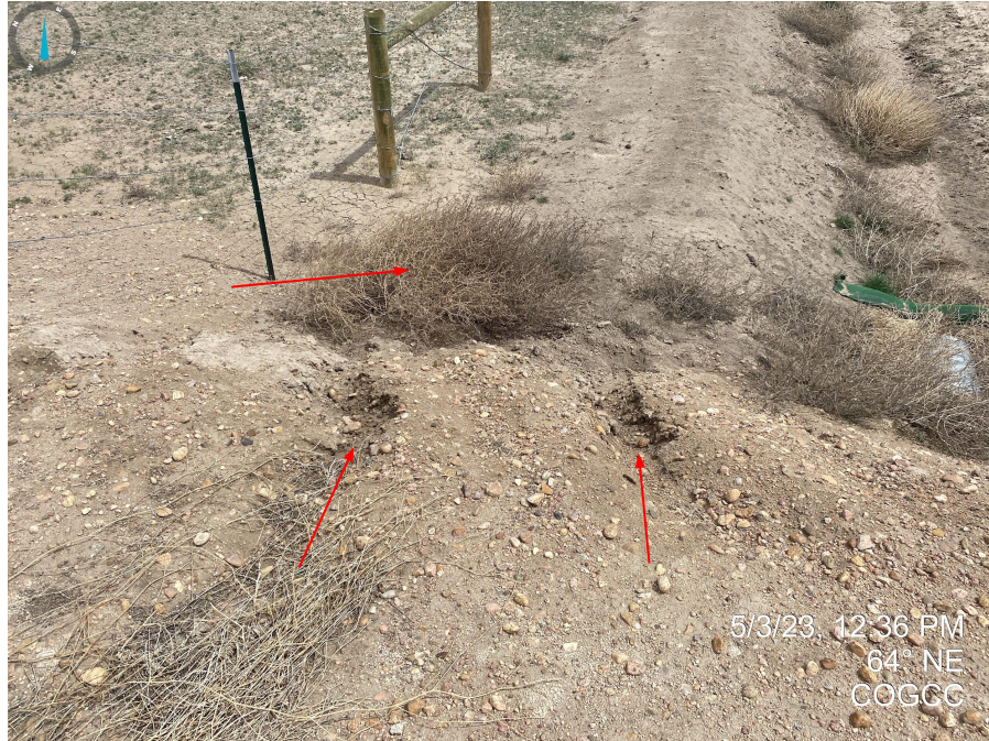
Photos 1 & 2. Rill erosion is evident at the entrance to the location. The inlet/outlets of the culvert will need to be properly stabilized/protected to prevent further erosion from occurring. Also pictured, undesirable plant debris that will need to be removed and managed for during the next local growing season.
