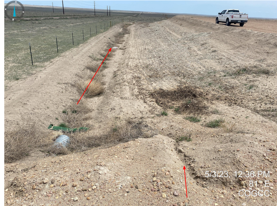
Photos 1 & 2. Rill erosion is evident at the entrance to the location. The inlet/outlets of the culvert will need to be properly stabilized/protected to prevent further erosion from occurring. Also pictured, undesirable plant debris that will need to be removed and managed for during the next local growing season.
