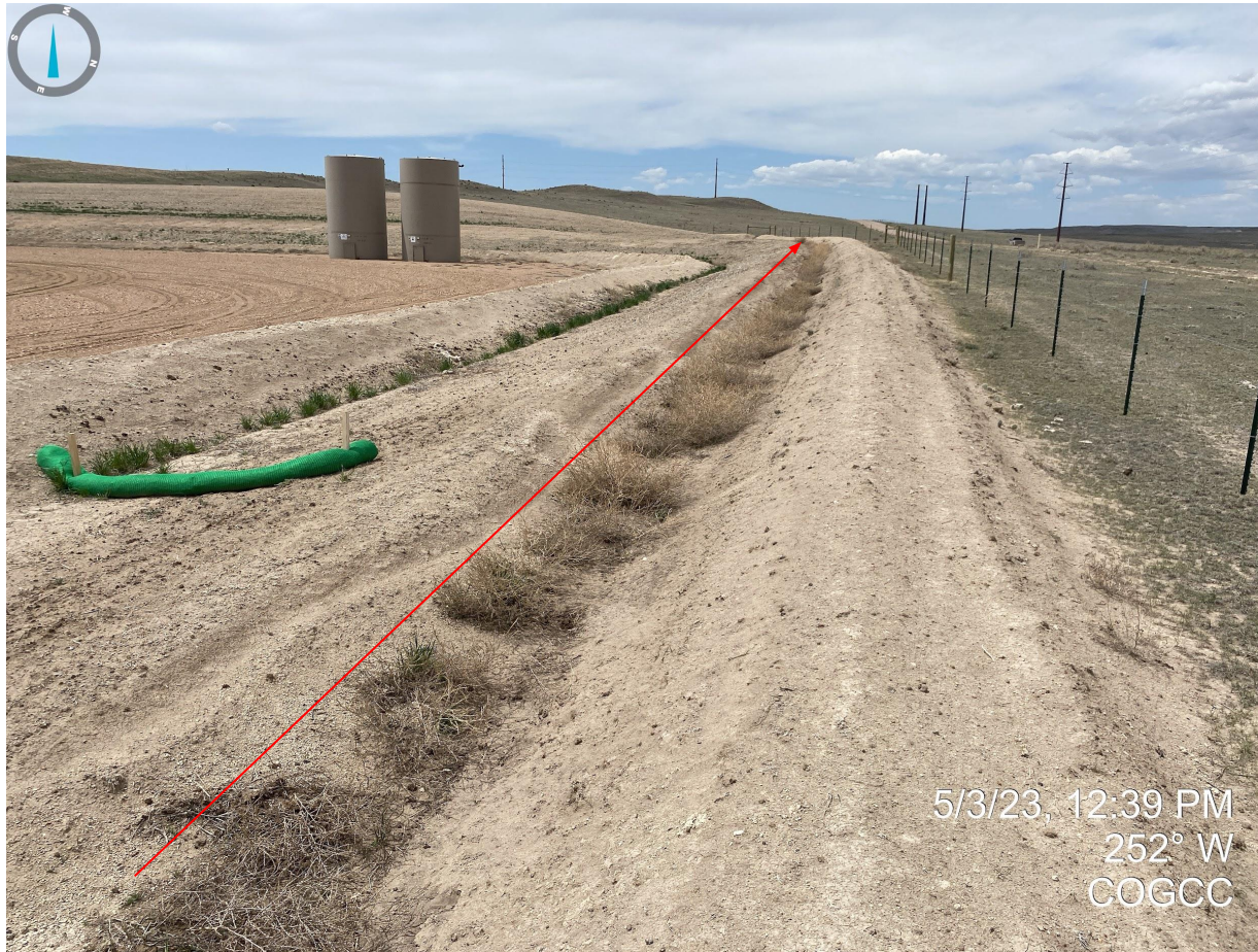
Photo 5. Undesirable vegetation in the ditch that does not appear to have been managed during the previous growing season.
