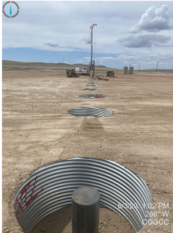
Photo 20. At the time of this inspection, cellars did not have any wildlife exclusion devices installed.
