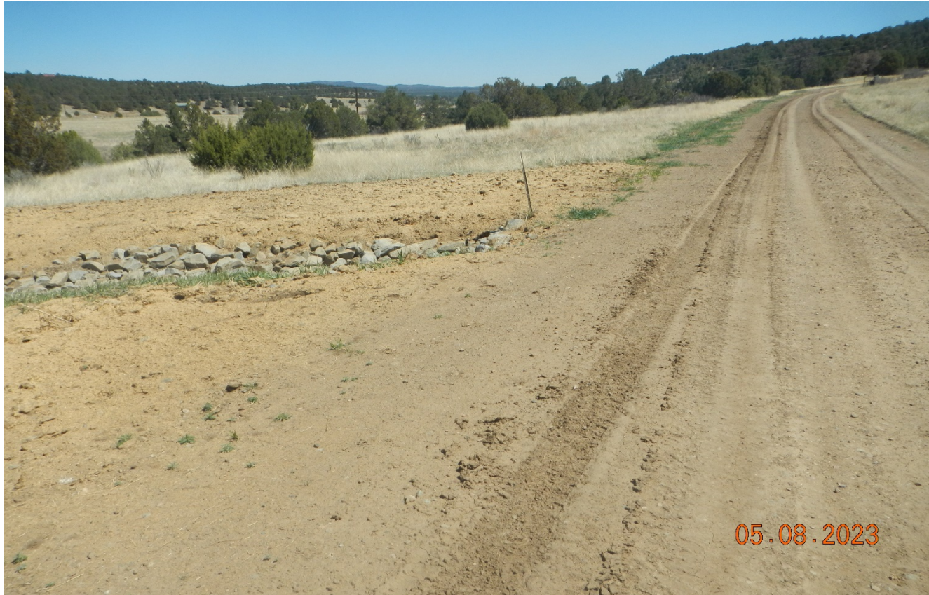
Photo 1. Facing northeast along the road. Culvert outlet protection was installed a disturbed areas were seeded and hydromulched.
