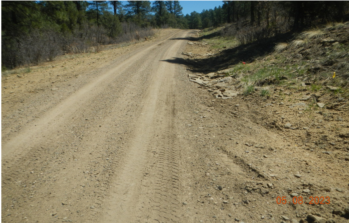
Photo 2. Facing northeast along the access road. Rock check dams were installed along the road and disturbed areas were seeded and hydromulched.
