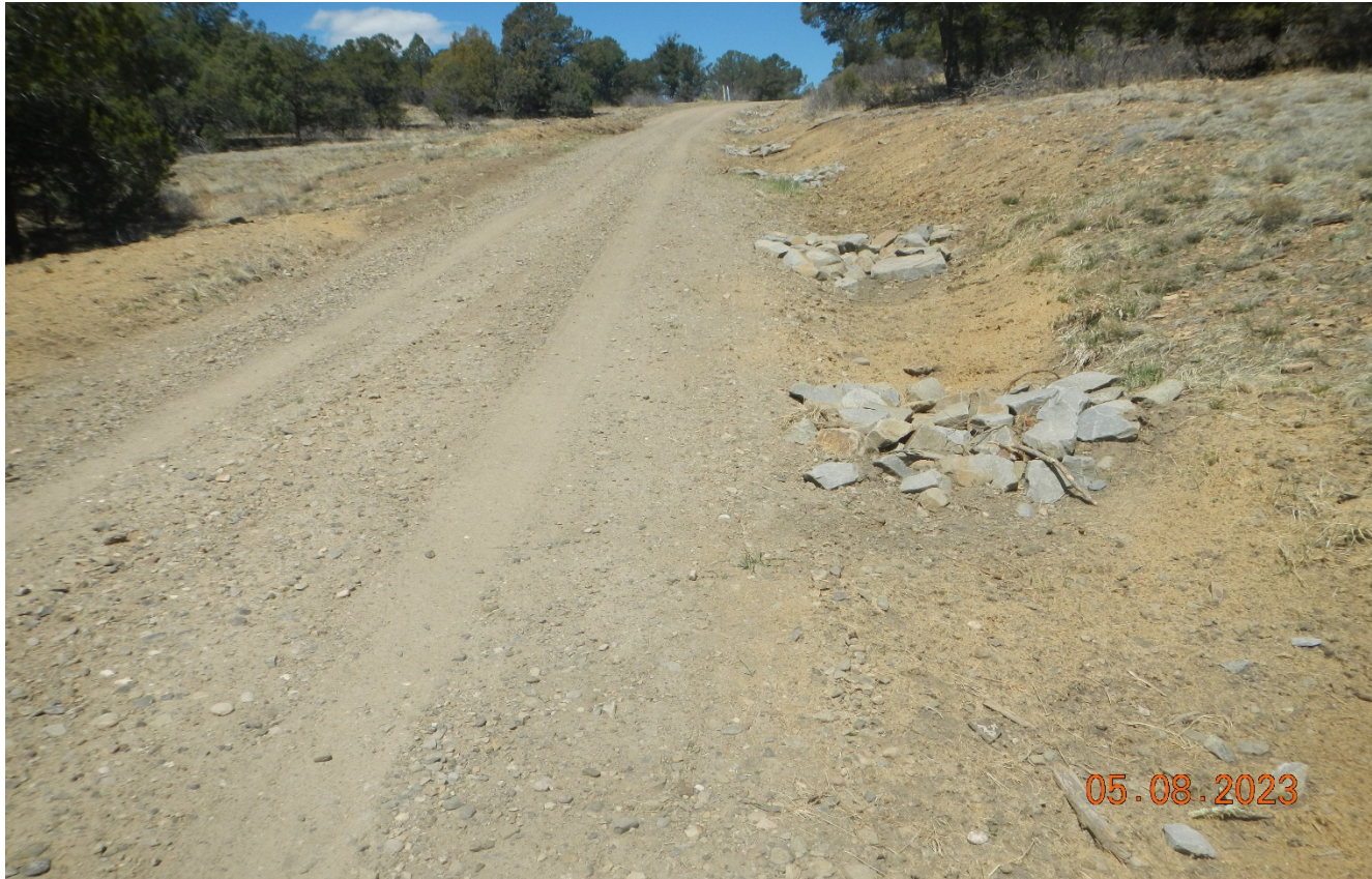
Photo 3. Facing north along the access road. Rock check dams were installed along the road and disturbed areas were seeded and hydromulched.
