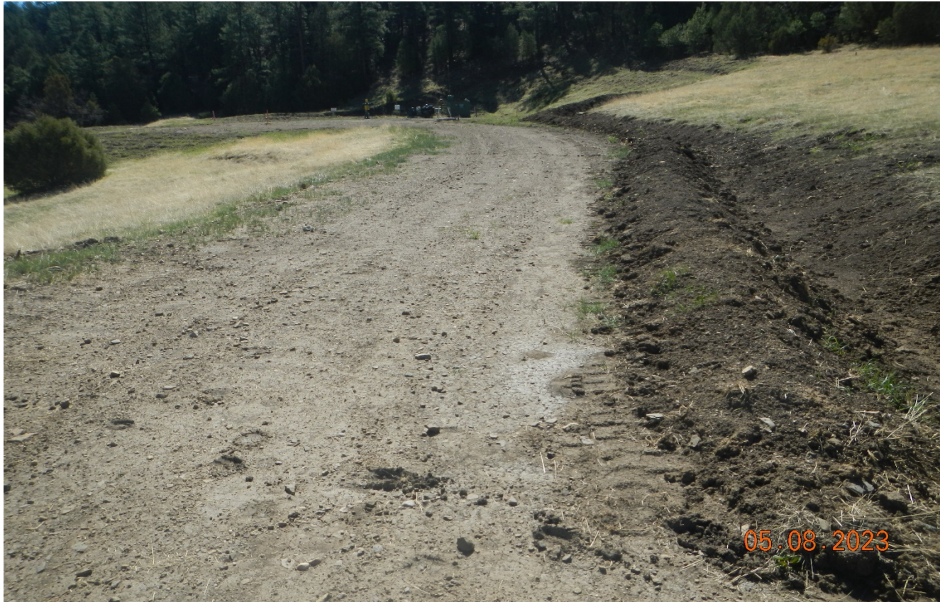
Photo 3. Facing southeast toward the wellsite. A diversion berm was installed along the road to the culvert.
