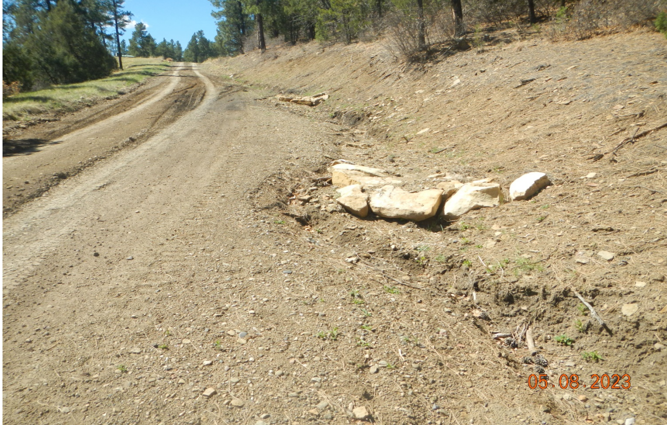
Photo 3. There is erosion is occurring around the rock check dams which has not been repaired since previous inspection.
