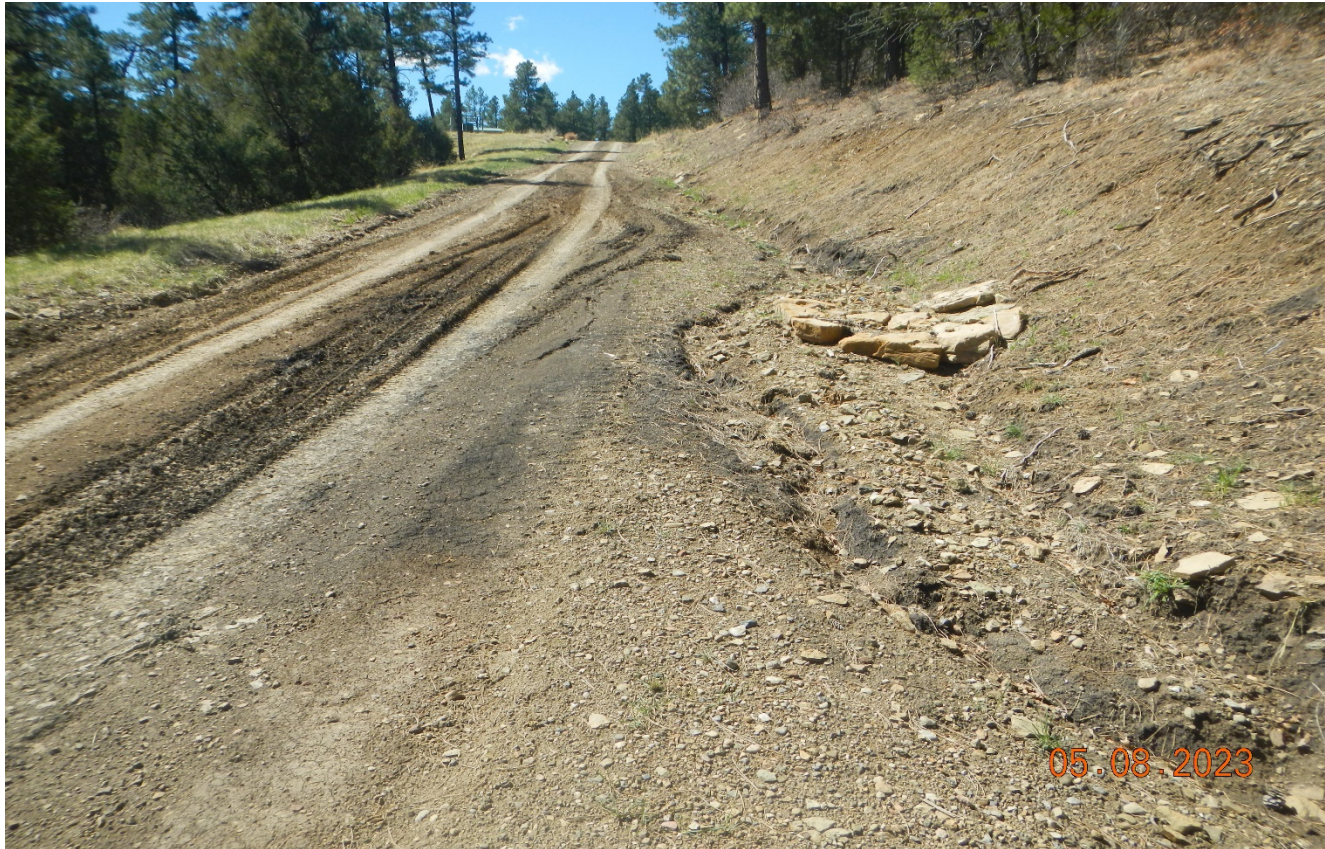
Photo 4. There is erosion is occurring around the rock check dams which has not been repaired since previous inspection.
