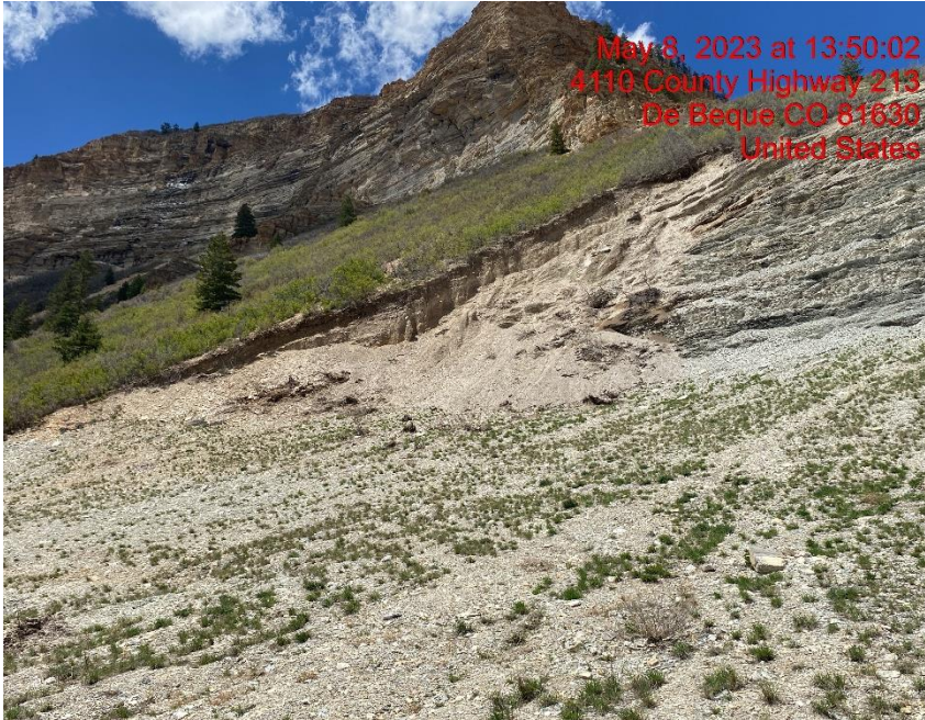
Cut Slope Eroding onto Location – Photo #03022
