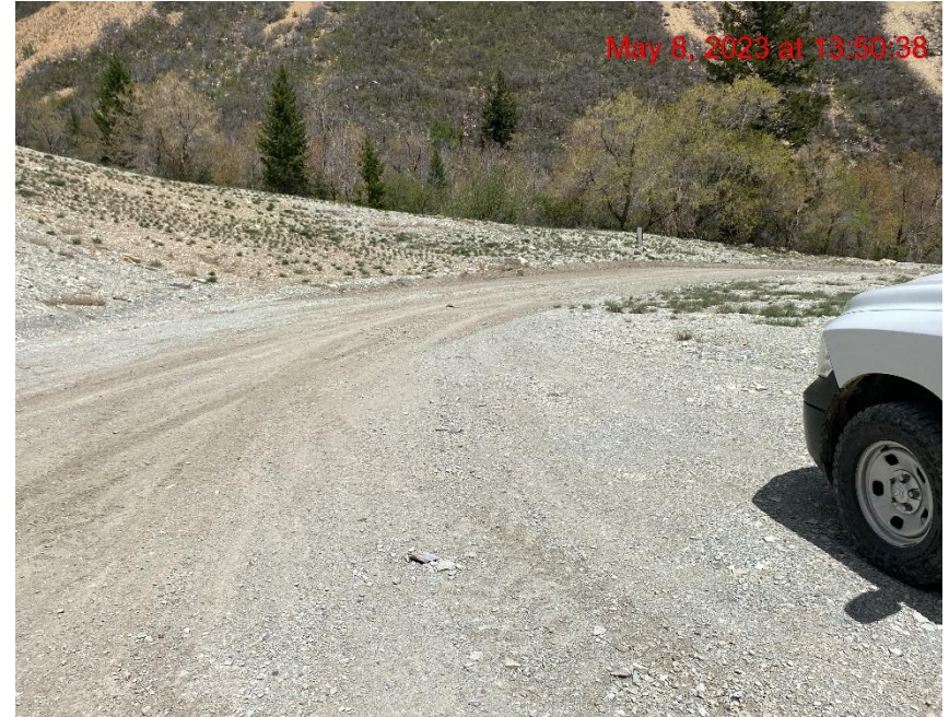
Insufficient Vehicle Tracking BMPs at Location Entrance/Exit – Photo #03023
