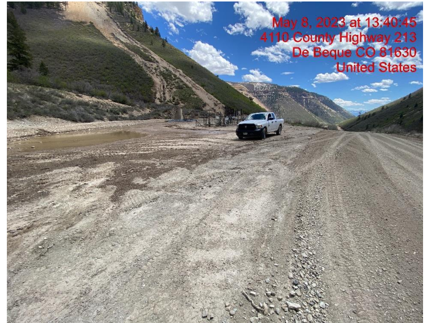
Insufficient Vehicle Tracking BMPs at Location Entrance/Exit – Photo #03006
