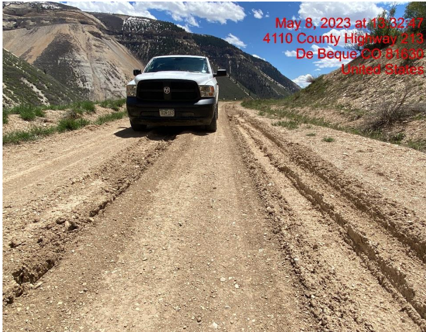
Lack of Stabilization on Access Road – Photo #02993
