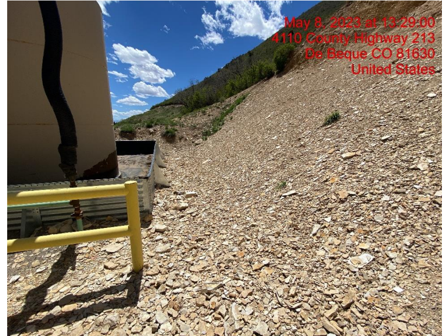
Cut Slope Eroding onto Location – Photo #02988
