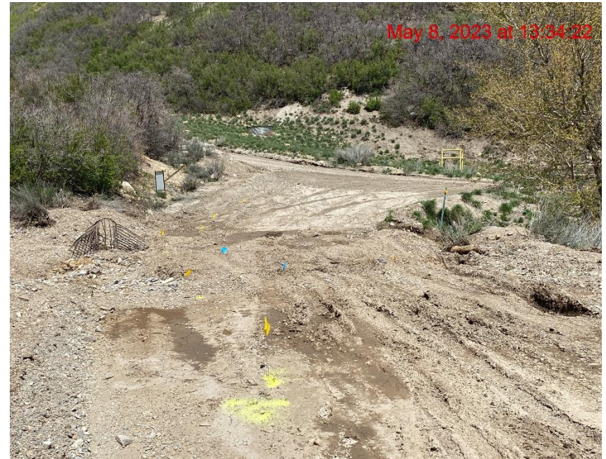
Insufficient Vehicle Tracking BMPs at Location Entrance/Exit – Photo #02994
