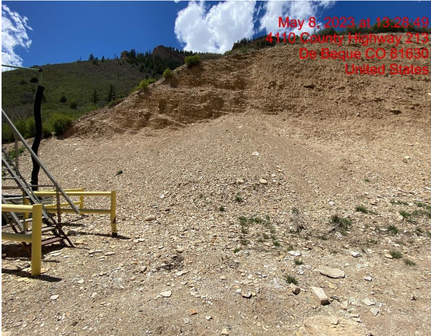
Cut Slope Eroding onto Location – Photo #02987
