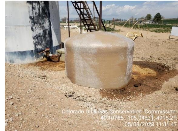
**Photo 13 Stained soil around the PW Tank inside berm.**
