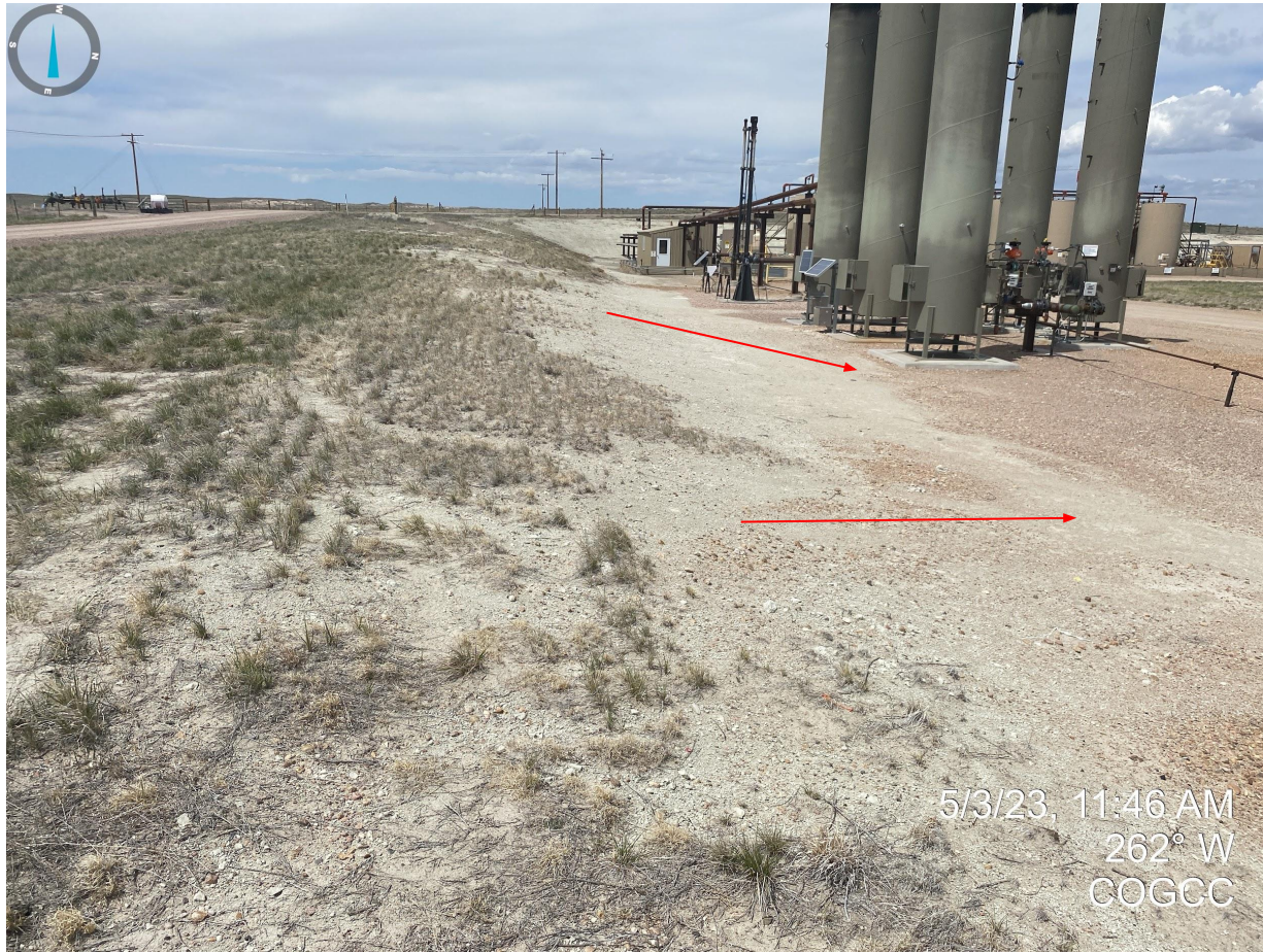
Photo 1. Southern portion of the production area. Photo illustrates that the cut slopes do not appear to be properly stabilized with non-uniform vegetation cover and evidence of sediment deposition into the production area. No apparent stormwater BMPs were observed to be implemented in these unstabilized areas.
