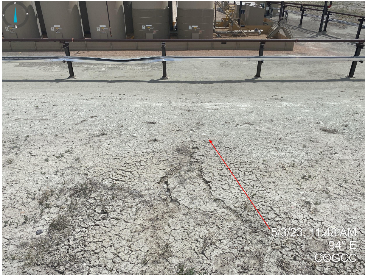
Photo 5. Rill erosion occurring on the unstabilized cut bank. Other than a perimeter stormwater ditch, no other stormwater BMPs were observed in this area.
