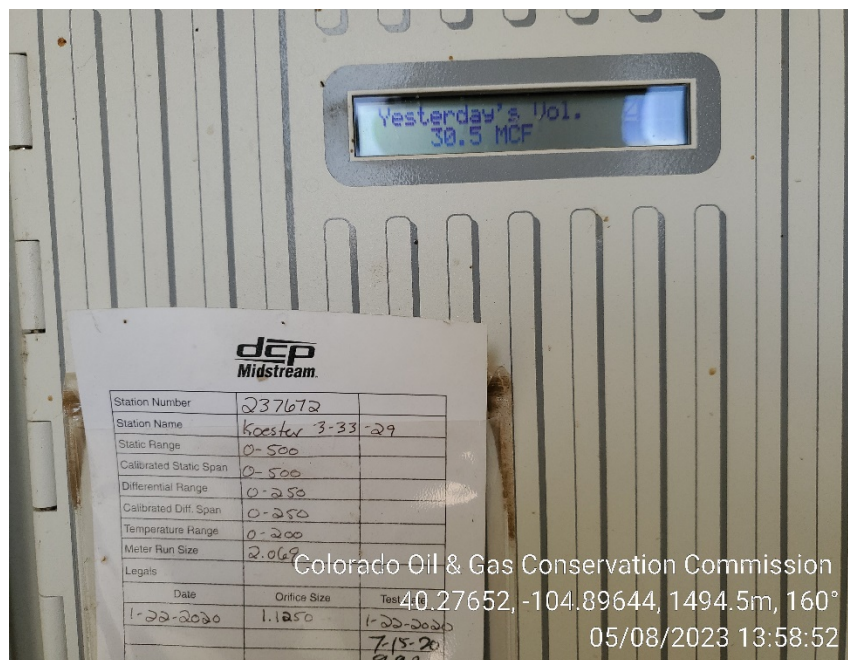
DCP gas sales meter calibration card and previous day product sold volume.
