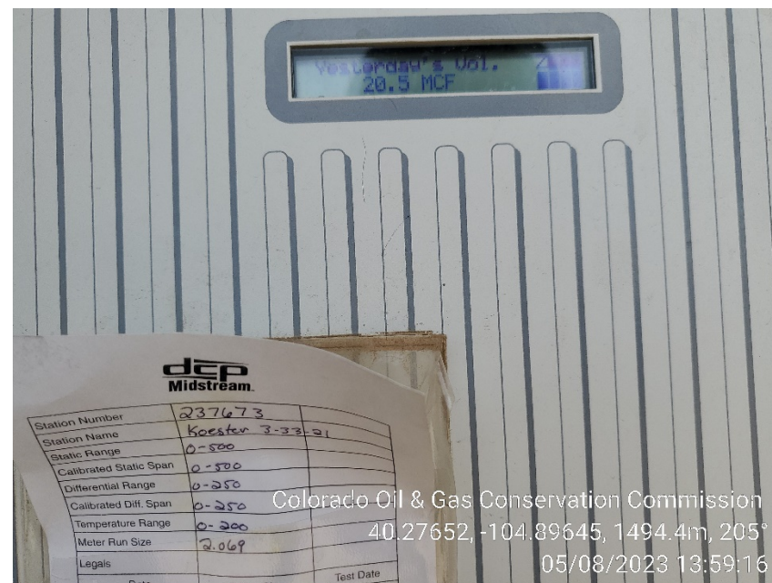
DCP gas sales meter calibration card and previous day product sold volume.
