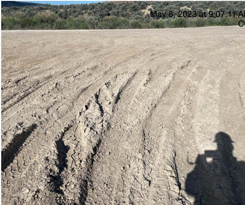
Photo # 7156 Lack of stabilization/compaction
