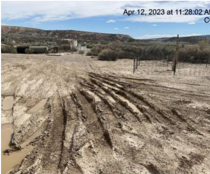
Photo # 5074 From Inspection 708900279 conducted on 04/12/2023 Lack of stabilization/compaction
