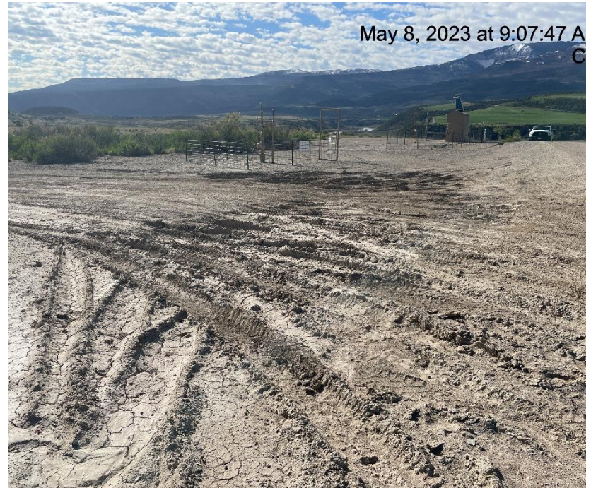
Photo # 7159 Lack of stabilization/compaction
