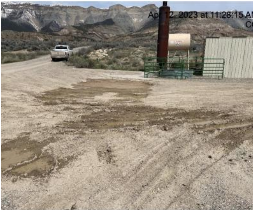
Photo # 5075 From Inspection 708900279 conducted on 04/12/2023 Lack of stabilization/compaction
