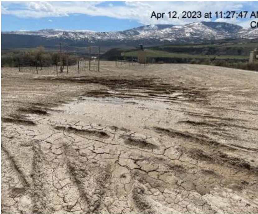
Photo # 5073 From Inspection 708900279 conducted on 04/12/2023 Lack of stabilization/compaction
