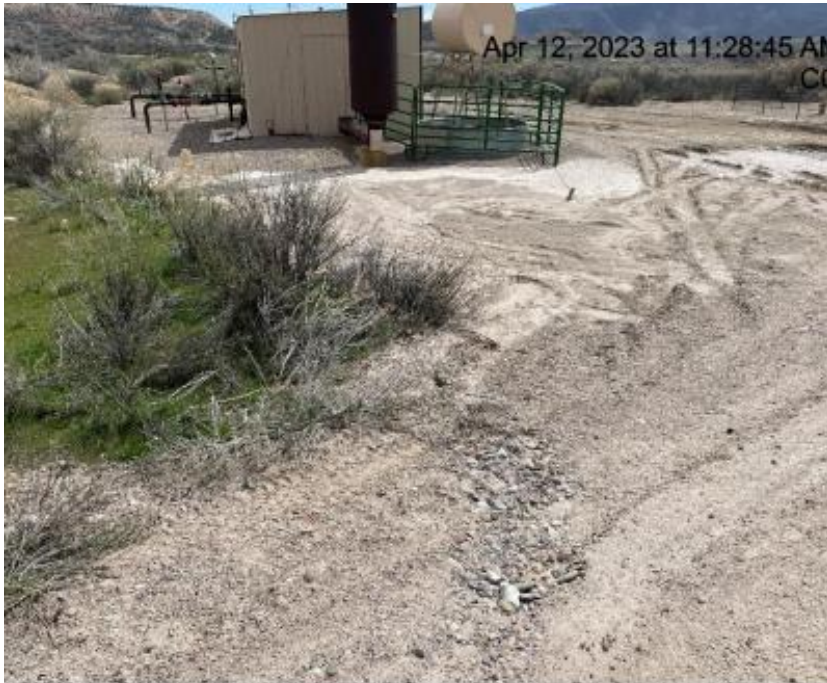
Photo # 5076 From Inspection 708900279 conducted on 04/12/2023 Erosion & transport of sediment onto location
