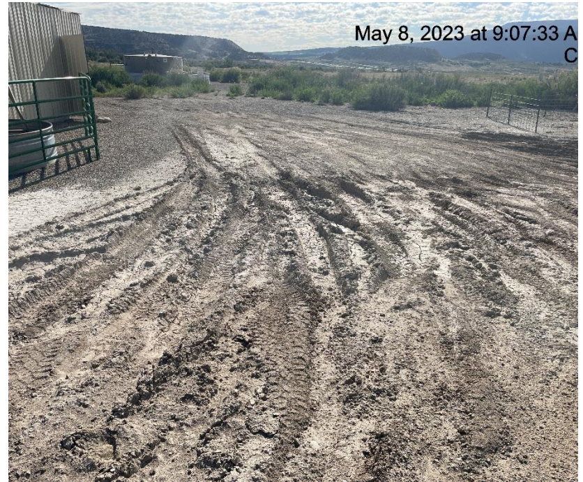
Photo # 7157 Lack of stabilization/compaction
