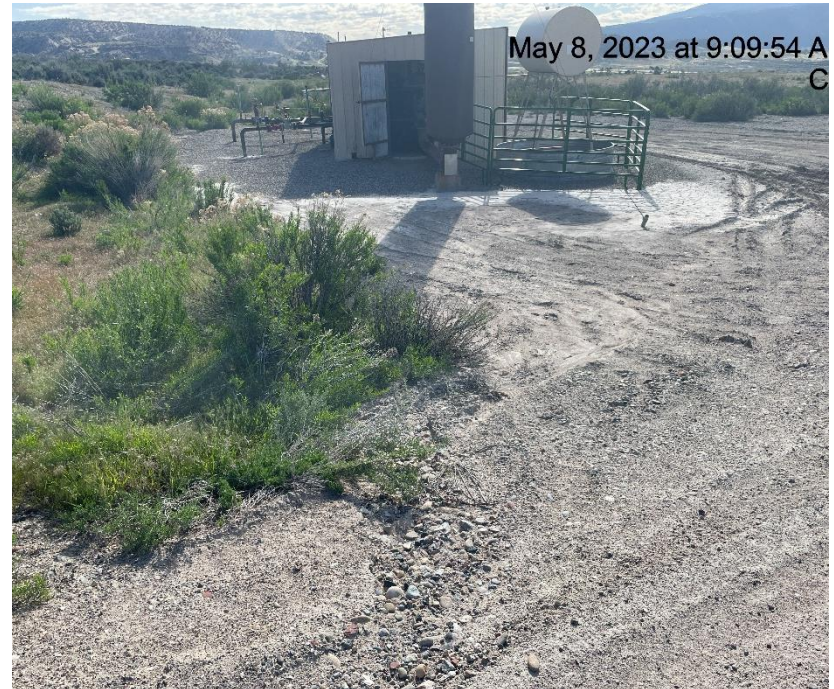
Photo # 7166 Erosion & transport of sediment onto location
