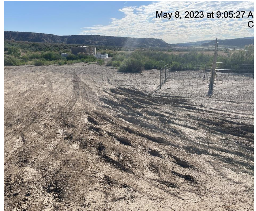
Photo # 7152 Lack of stabilization/compaction
