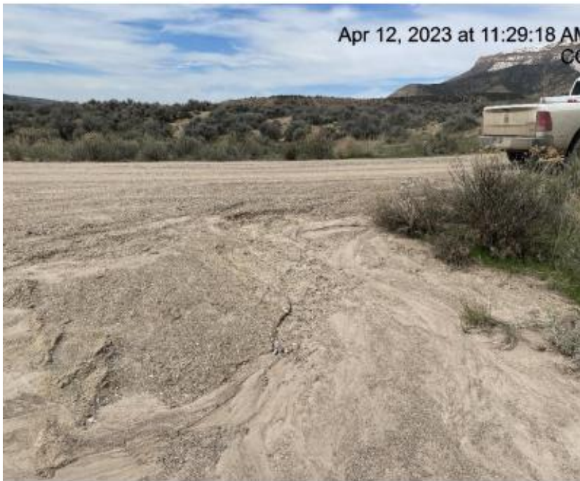
Photo # 5079 From Inspection 708900279 conducted on 04/12/2023 Erosion & transport of sediment onto location
