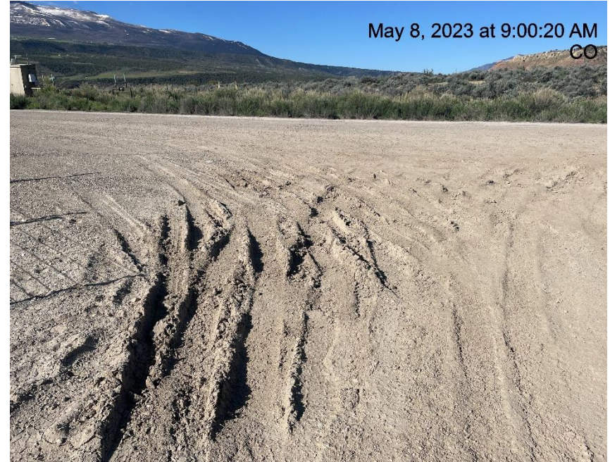
Photo # 7145 Lack of stabilization/compaction
