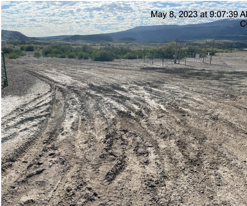
Photo # 7158 Lack of stabilization/compaction
