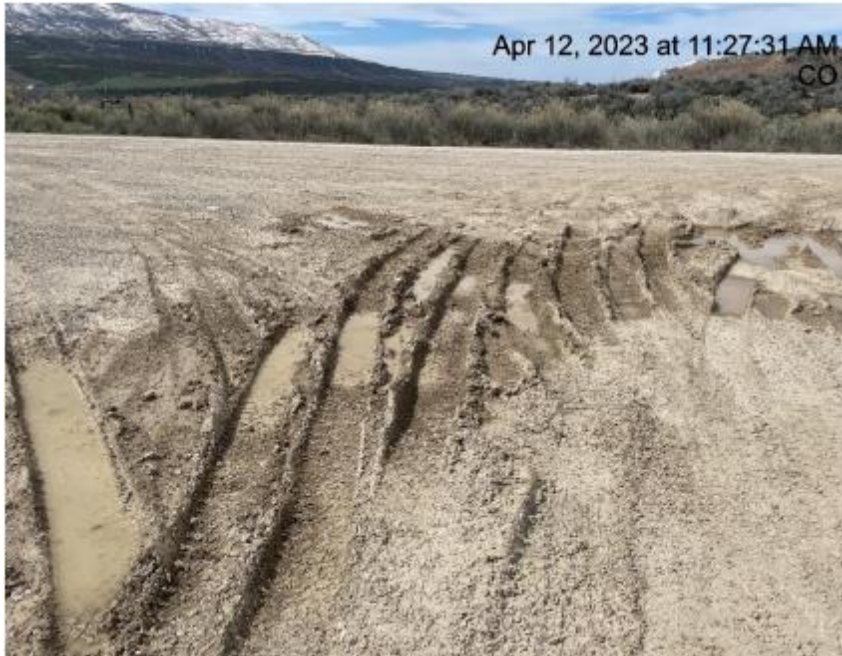
Photo # 5072 From Inspection 708900279 conducted on 04/12/2023 Lack of stabilization/compaction
