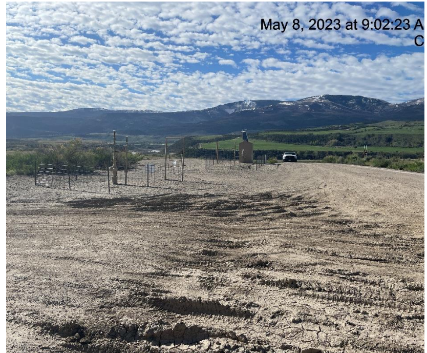
Photo # 7148 Lack of stabilization/compaction
