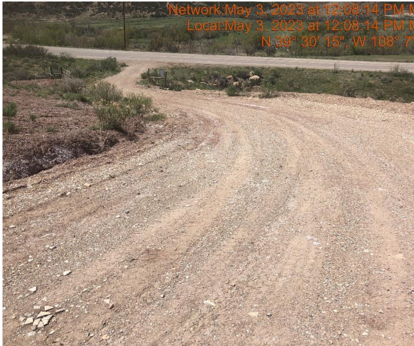
Photo #9831 Insufficient tracking BMP at entrance to location.
