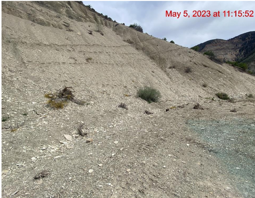
Cut Slope Eroding onto Location – Photo #02945
