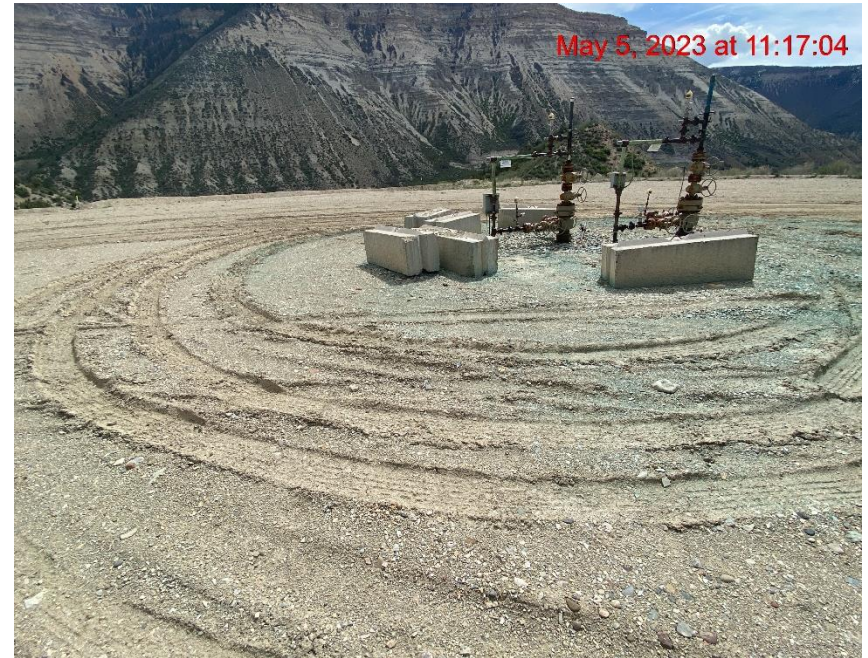
Location Lacks Stabilization – Photo #02949
