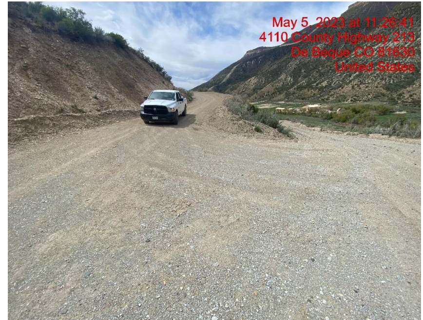
Insufficient Tracking BMPs at Location Entrance/Exit – Photo #02959
