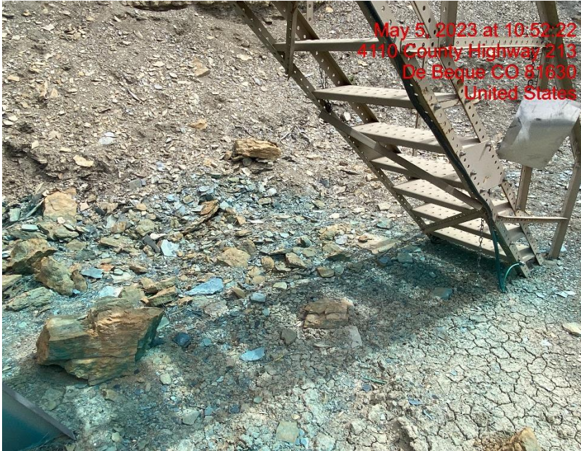
Cut Slope Eroding into Production Equipment – Photo #02917
