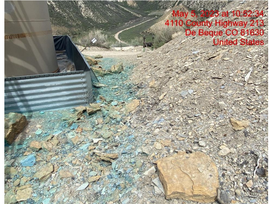
Cut Slope Eroding into Production Equipment – Photo #02918
