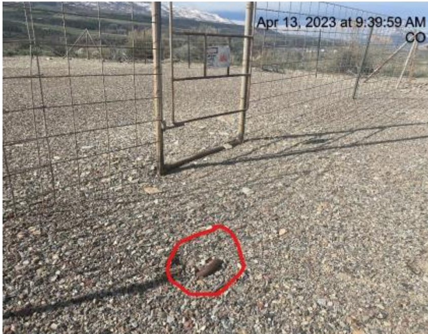
Photo # 5333 From Inspection 708900277 conducted on 04/13/2023 Unmarked deadman
