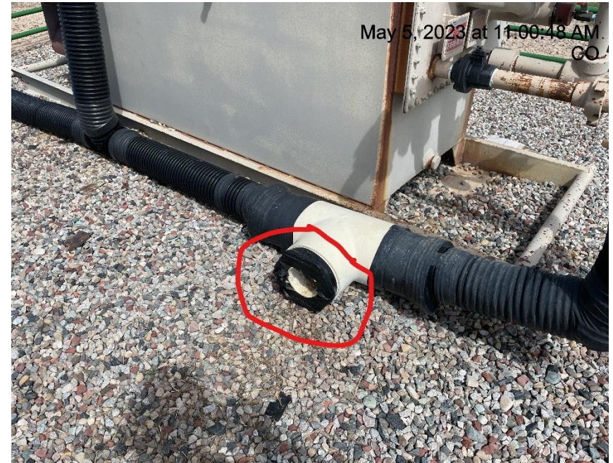
Photo # 7043 Flow line heating insulation open ended/wildlife hazard
