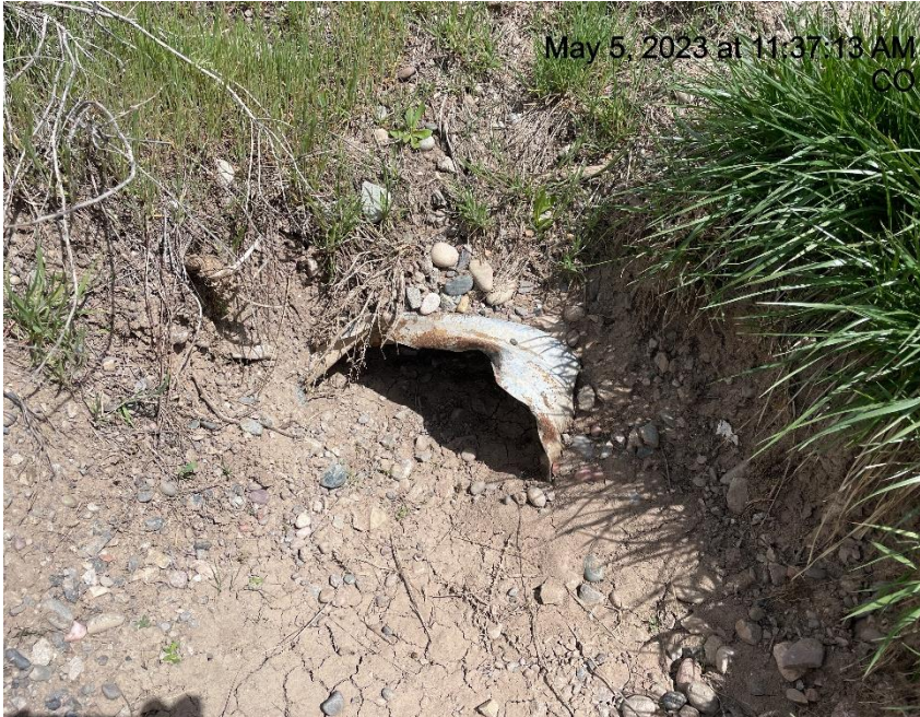
Photo # 7132 Culvert needs maintenance (Culvert is located at the start of the access road right before the gates)
