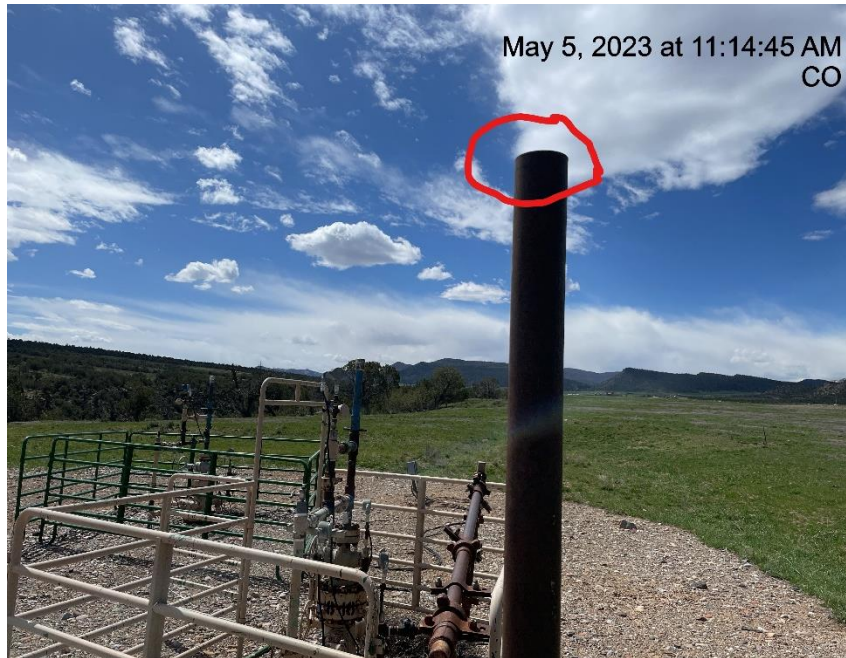
Photo # 7063 Open ended piping/wildlife hazard
